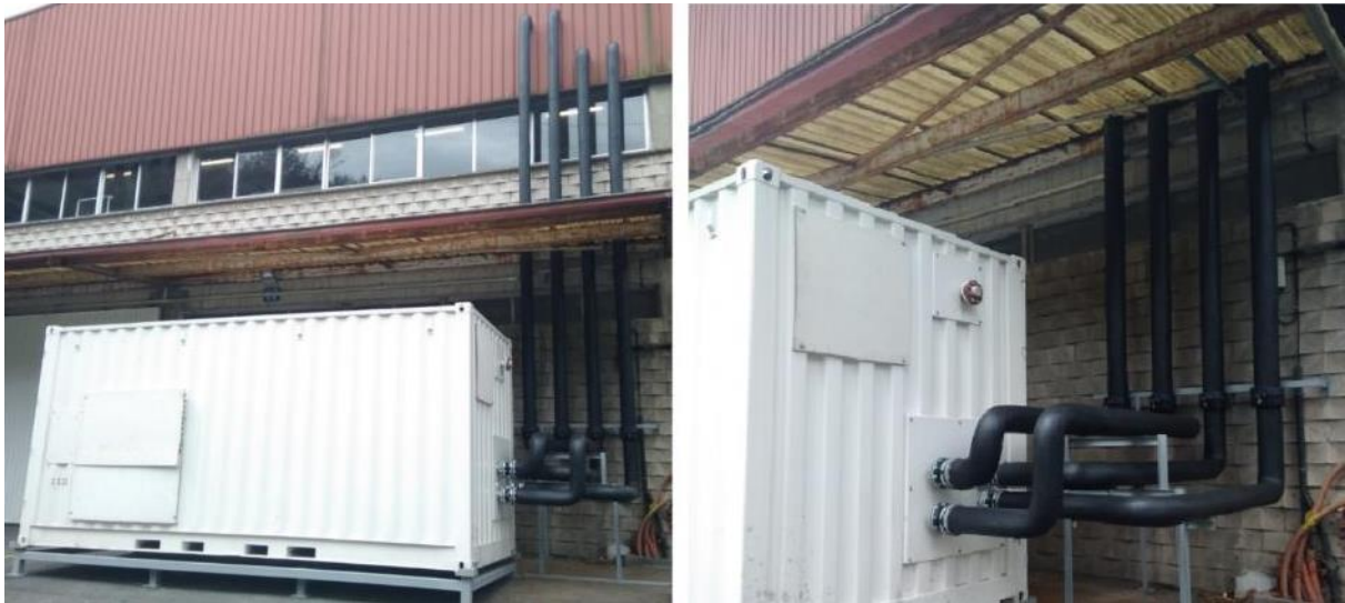
Figure 49. Pipes with final insulation
