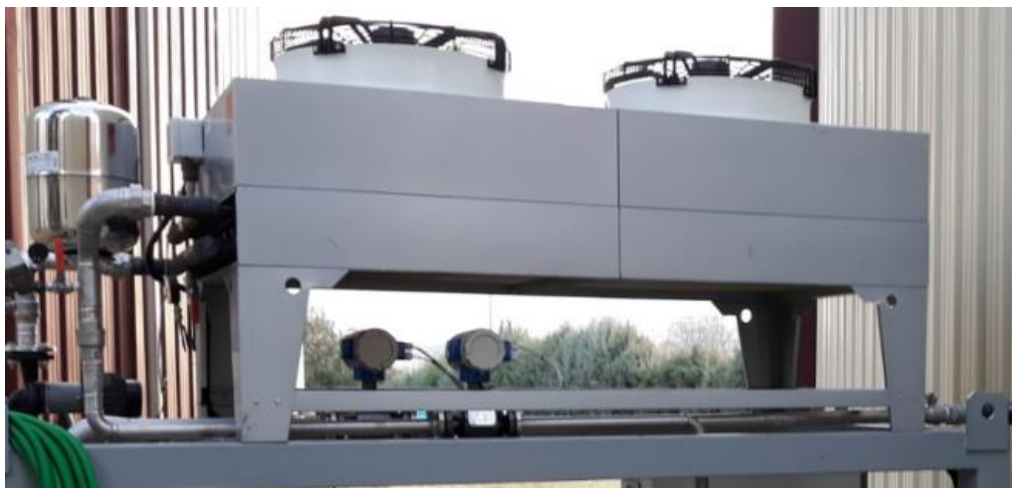
Figure 8. Dry cooler at Madrid WWTP
