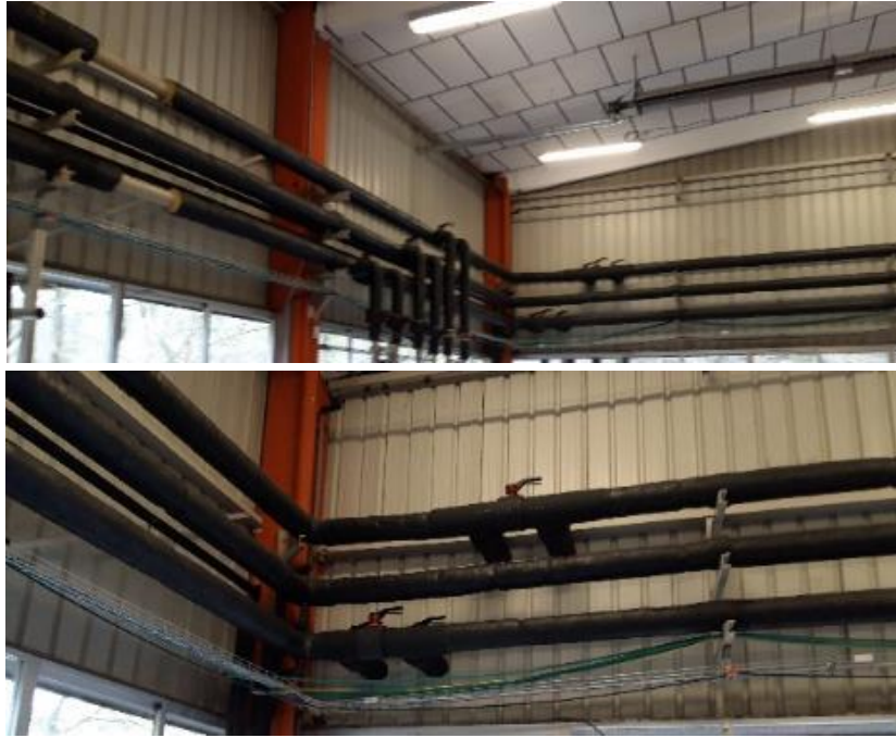
Figure 51. Distribution loops for heat generation and rejection
