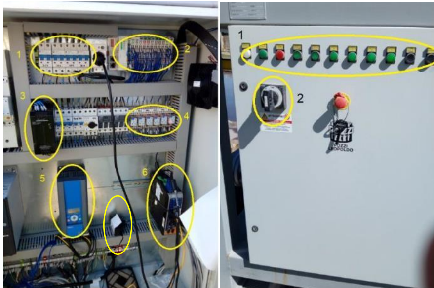
Figure 32. Inside components of the cabinet (left) and outside components (right); Status information lights (1) and Circuit breaker (2)
