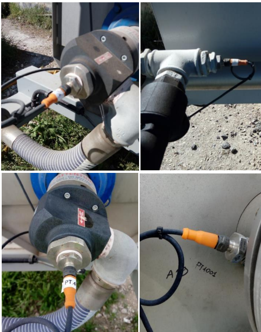
Figure 28. Temperature sensors
