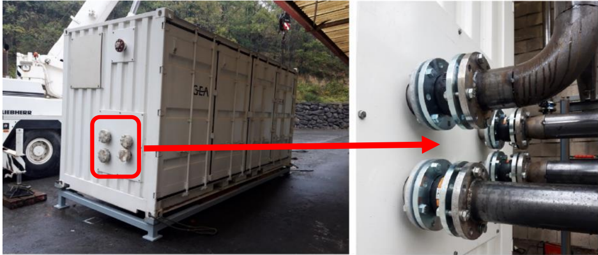
Figure 47. Connection with containerized Heat Pump
