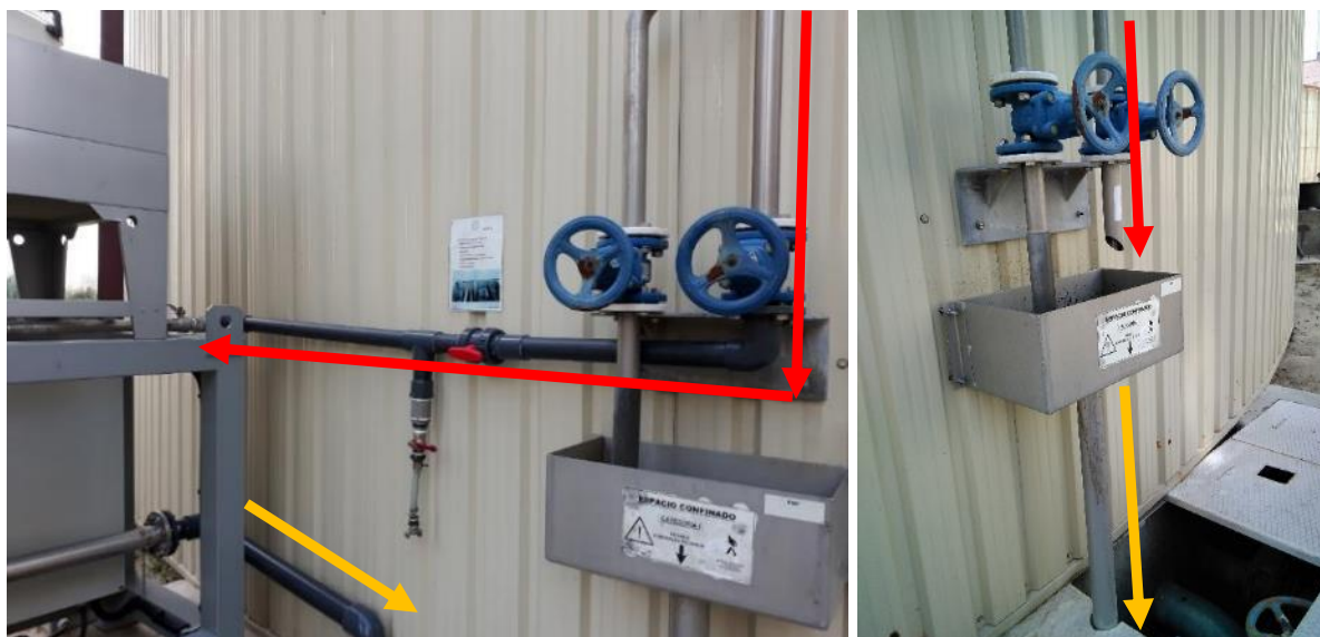
Figure 18: Integration of modified sludge pipe with the RHeX unit
