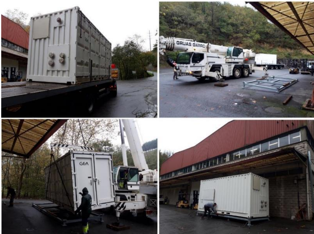
Figure 45. Discharge and placement of GEA Heat Pump
