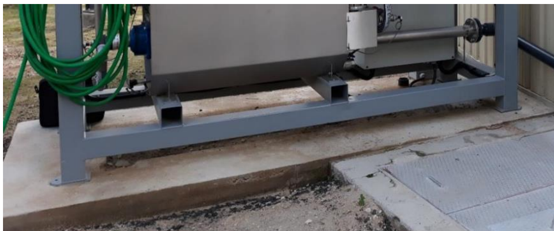
Figure 15: Foundation slab for skid levelling
