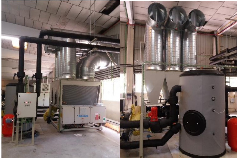
Figure 52. Daikin chiller (left) with primary loop and storage tank (right)
