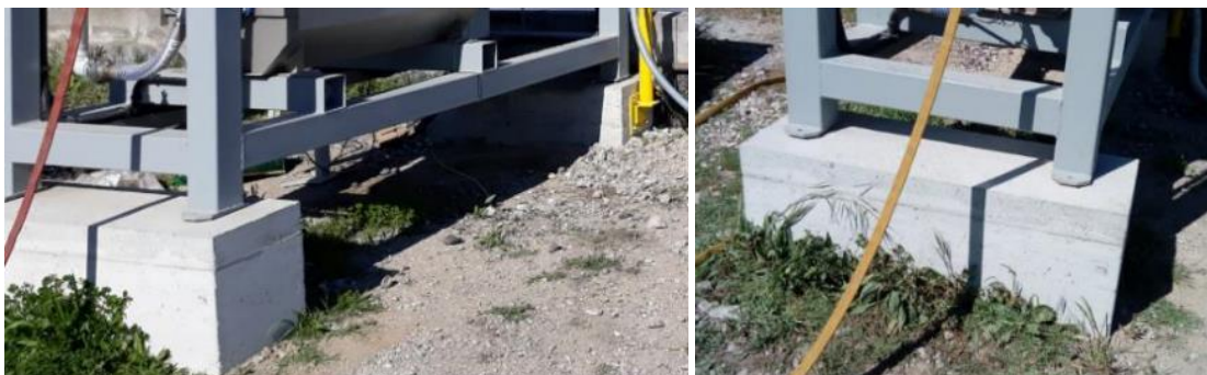
Figure 33. Blocks holding skid
