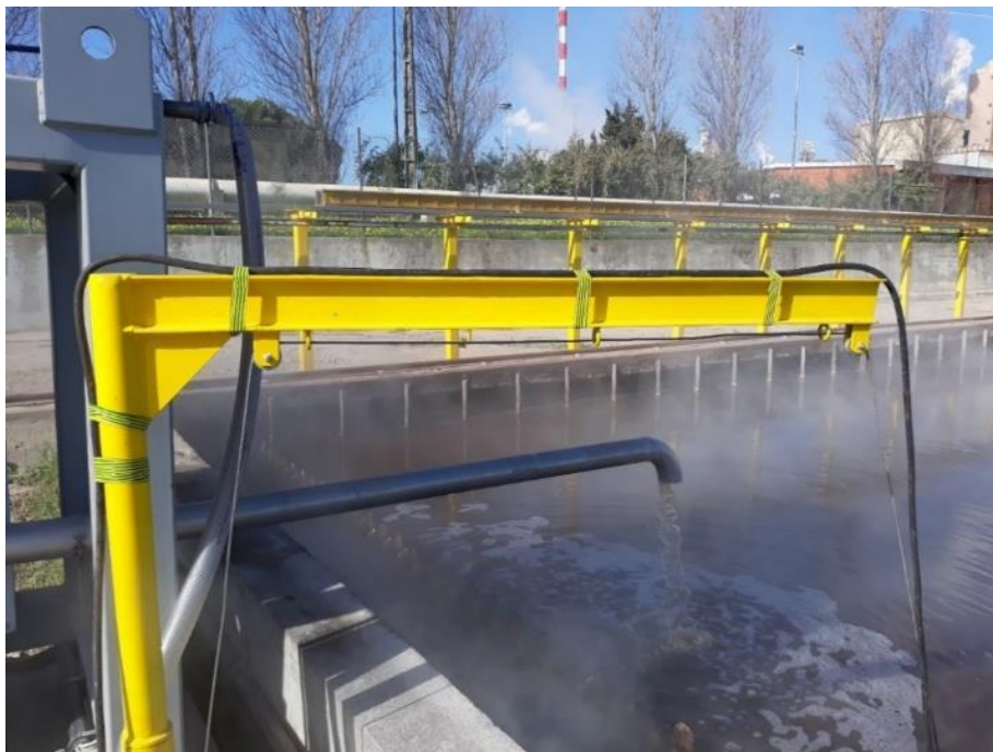
Figure 35. The mechanism to keep the pump in an upright position and effluent return to the pool
