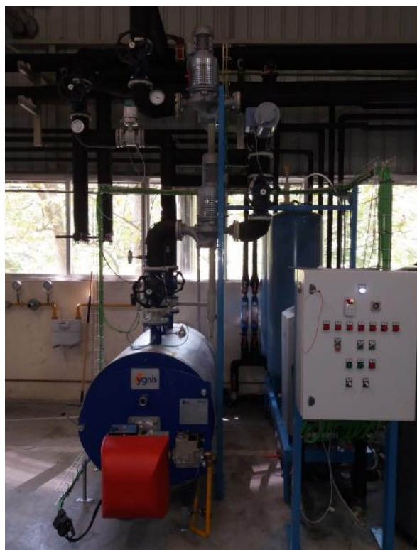
Figure 54. Heat input system and primary pump to the evaporator
