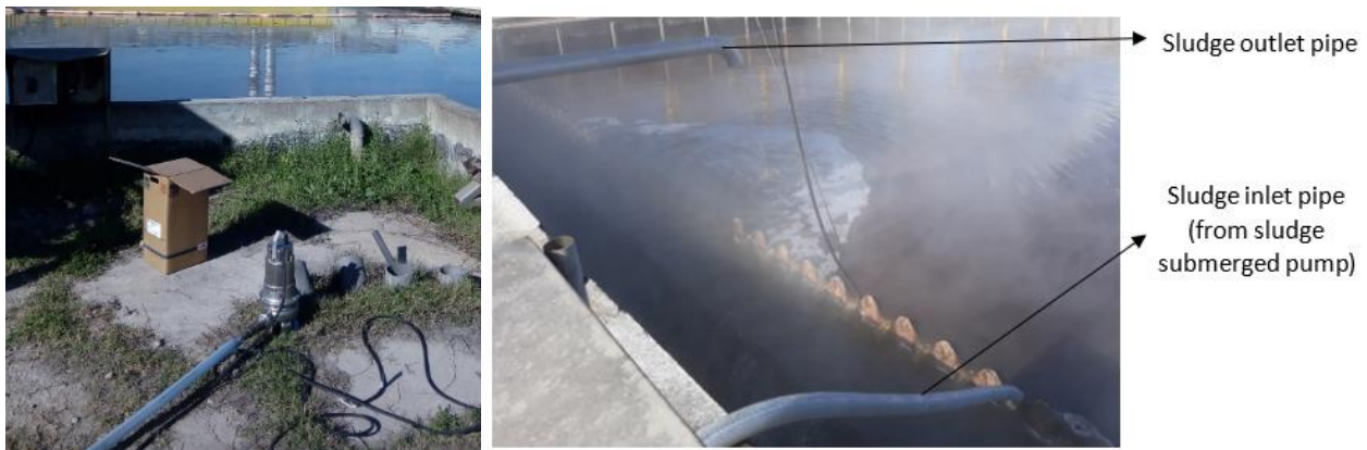
Figure 34. Sludge pump before (left) and after being submerged in the sludge with piping
