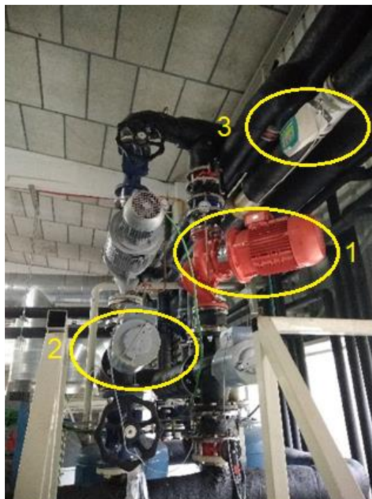
Figure 55. Heat loop pump to HP (1), three-way control valve (2) and flowmeter (3)
