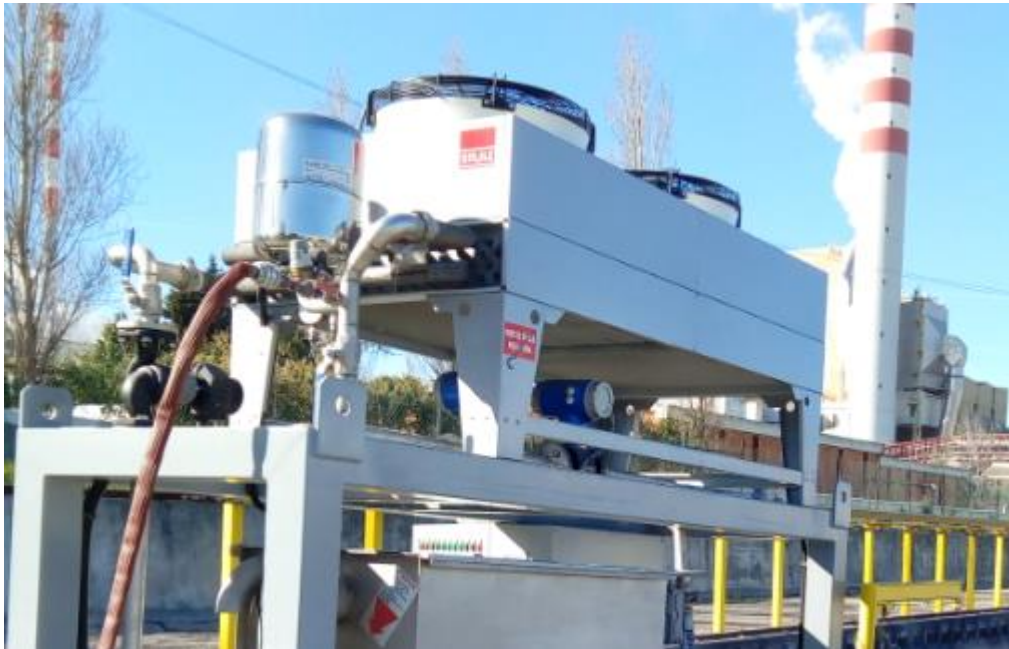
Figure 26. Dry cooler installed over the skid
