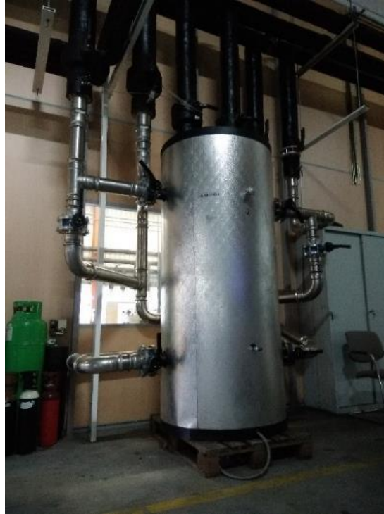
Figure 56. Premixed storage tank (1.000l)
