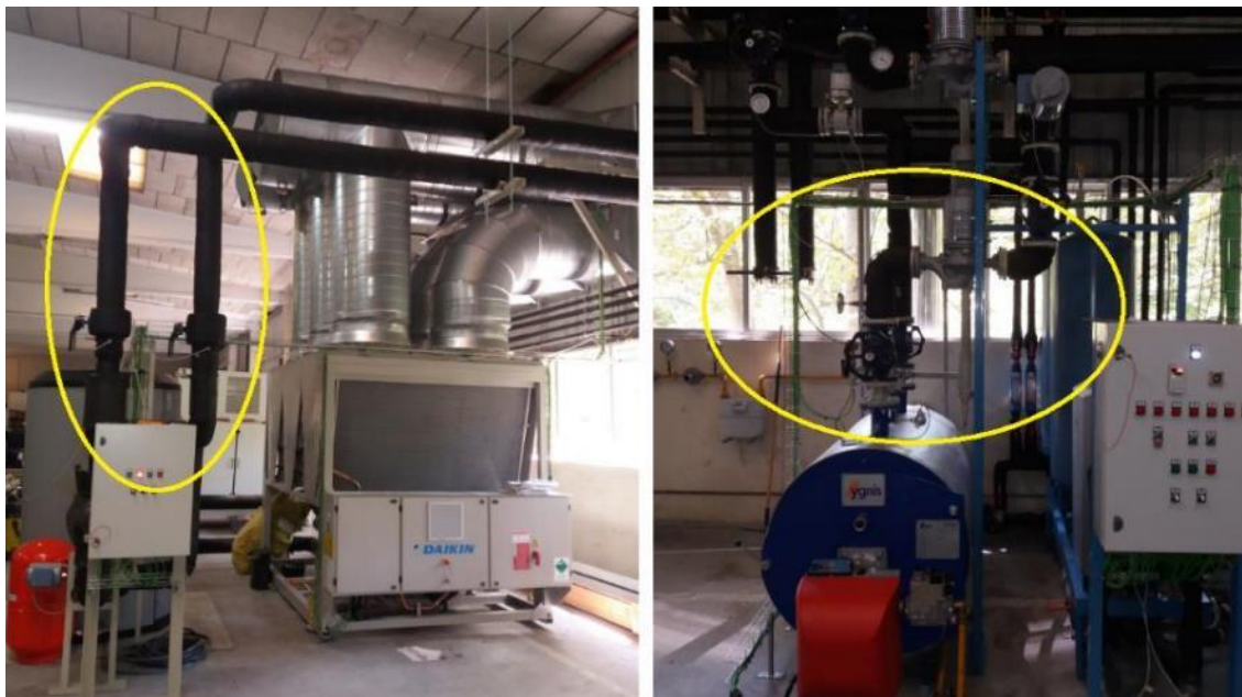
Figure 50. Pipes connection with the chiller (left) and pipes connection with boiler (right)
