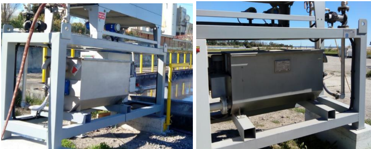
Figure 25. Heater exchanger installed
