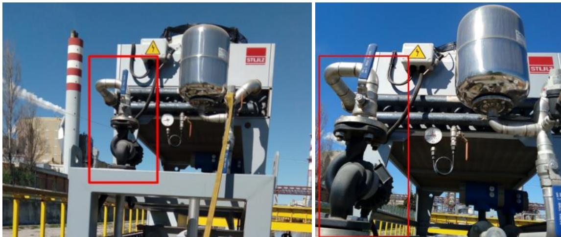
Figure 27. Water pump installed
