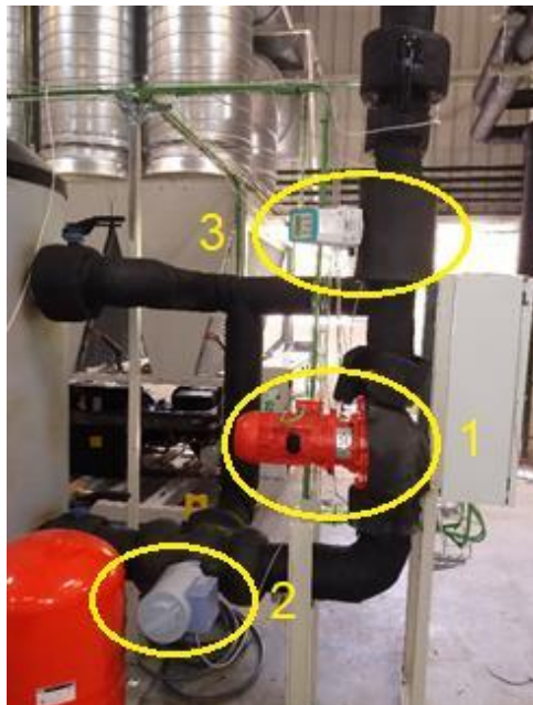
Figure 53. Pump (1), three-way valve with its control cabinet (2) and a flow meter (3)
