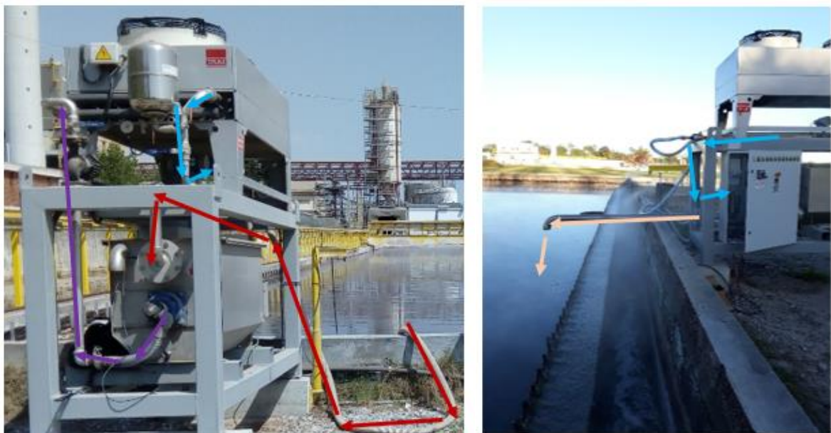
Figure 37. Operation scheme of LowUP system in Setubal demo site
