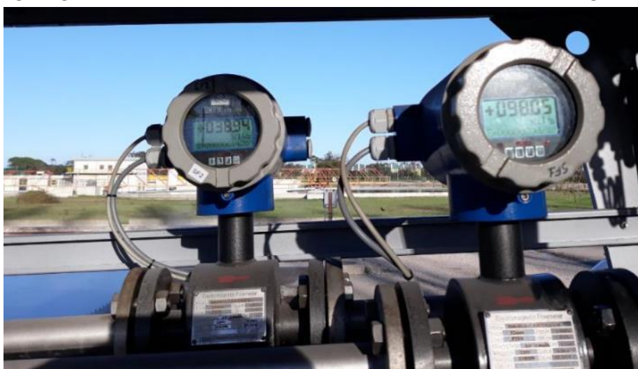
Figure 29. Two flow meters installed
