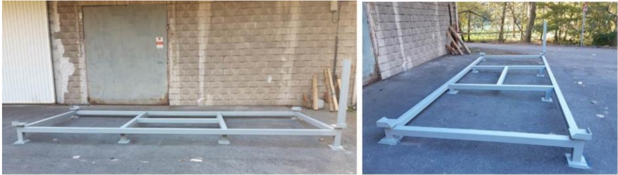
Figure 44. Bearing structure for the Heat Pump
