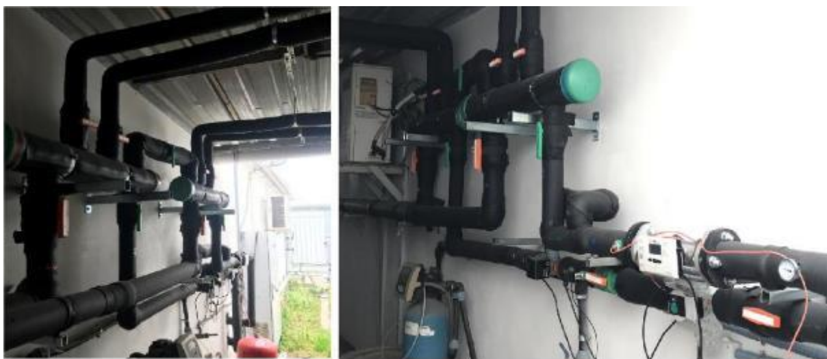
Figure 50. Radiant floor collector and piping connections
