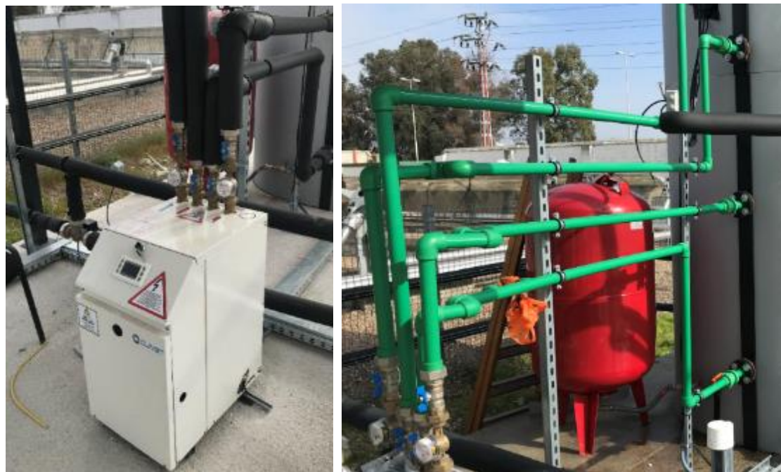
Figure 20. Heat pump and piping connections
