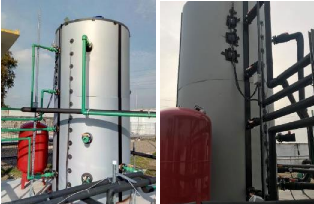
Figure 17. Stratified tank with connections
