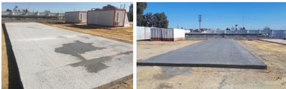
Figure 13. Foundation slab for PVT system.
