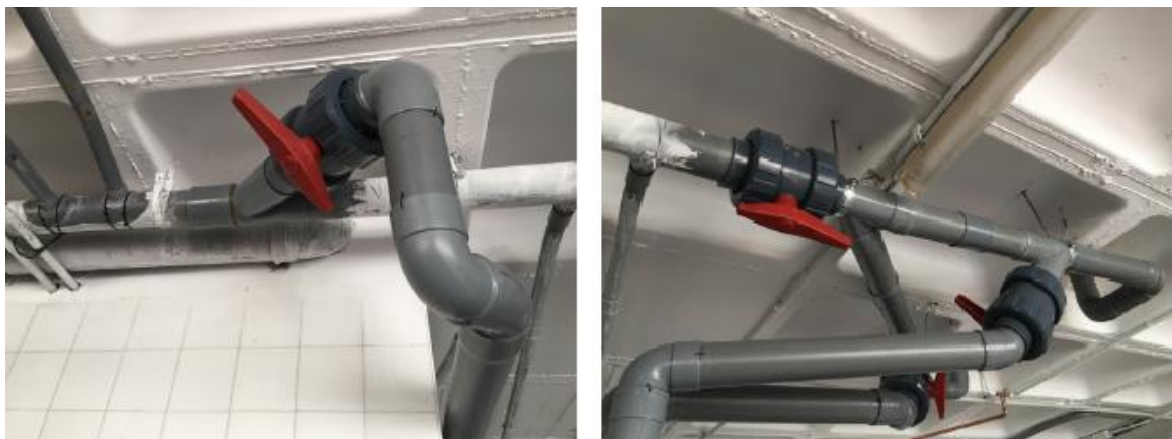
Figure 80. Details of new pipelines to HWHR for grey waters
