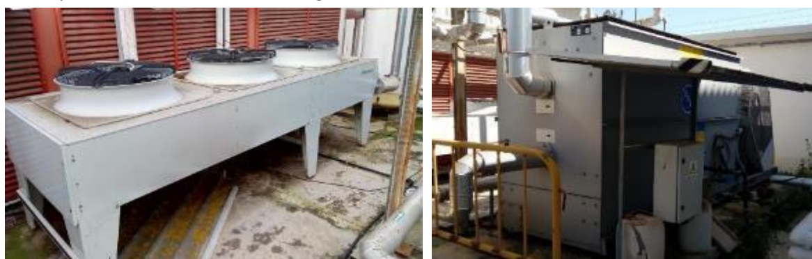
Figure 39. Dry cooler for emulation (left) and wet cooling tower for dissipation (right)
