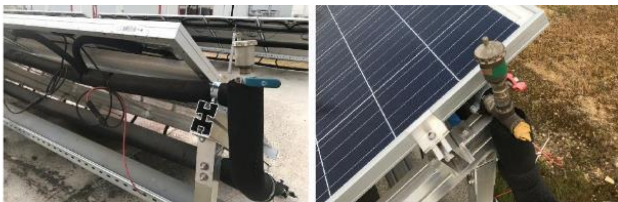
Figure 32. Bleeder distributed in the solar field
