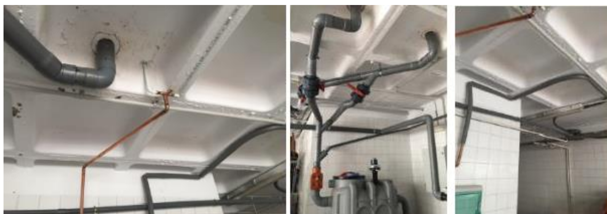
Figure 79. New pipelines to HWHR for grey and clean waters
