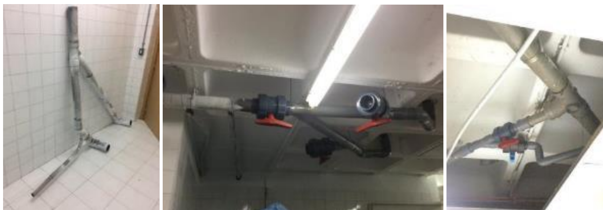
Figure 78. Replaced pipes (left), new pipes connections of the kitchen sinks (centre) and Item 3: Dishwasher 1 and 2 (right)
