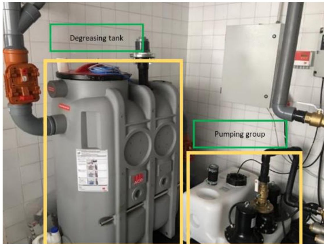
Figure 90. Inlet of grey waters
