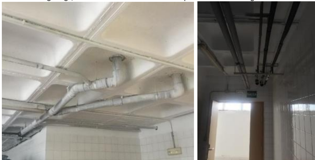
Figure 76: Current state of pipe system: grey waters (left) and clean water (right)
