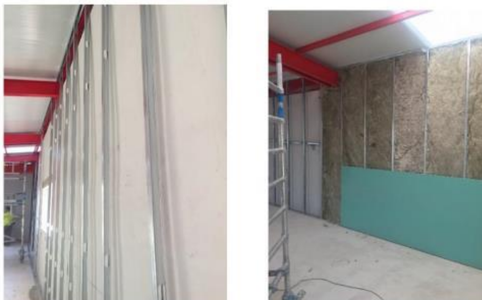
Figure 7. Insulation of the walls.
