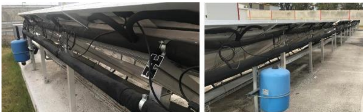
Figure 29. Backface of the PVT panel (Collector and expansion tank)
