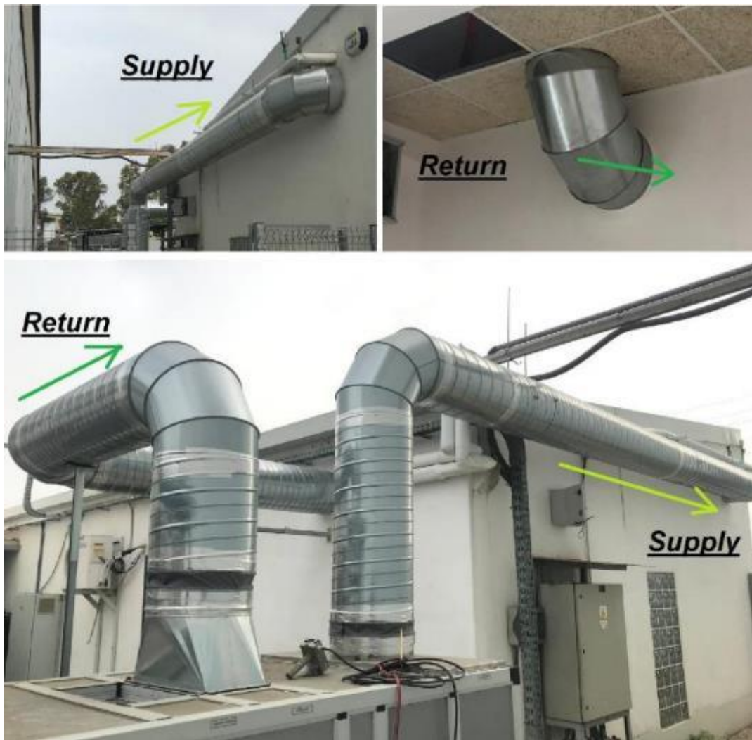
Figure 41. Supply and return duct of the AHU
