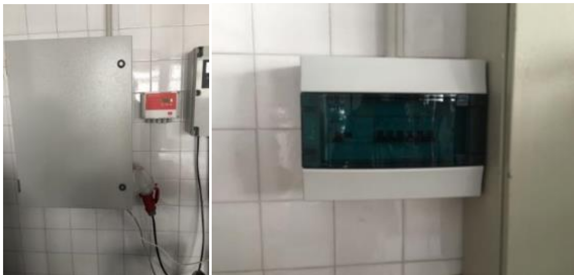
Figure 87. Cabinet of control and monitoring power supply (left) and power supply cabinet (right)
