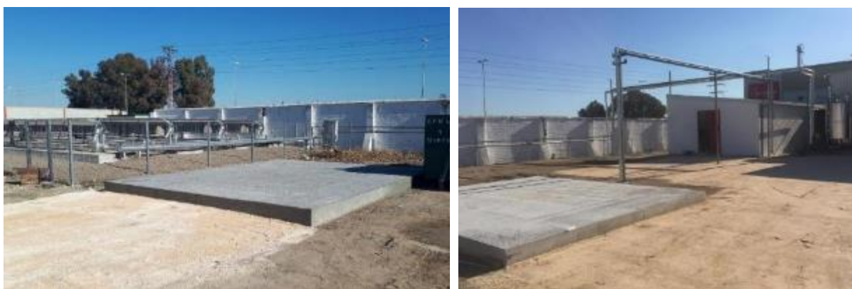
Figure 11. Foundation for stratified thermal storage installation
