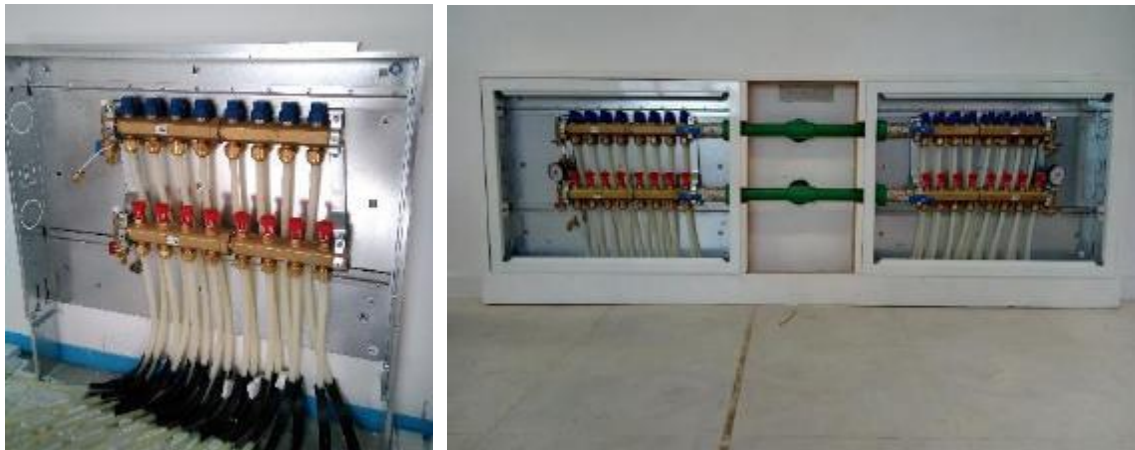
Figure 47. Manifolds of the radiant floor
