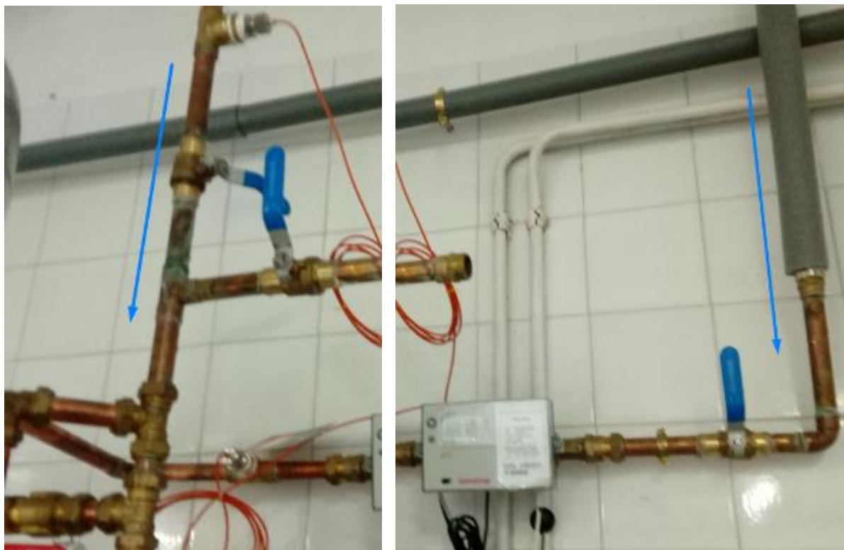
Figure 85. Coldwater inlet from the network (left) and pre-heated cold-water inlet (right)
