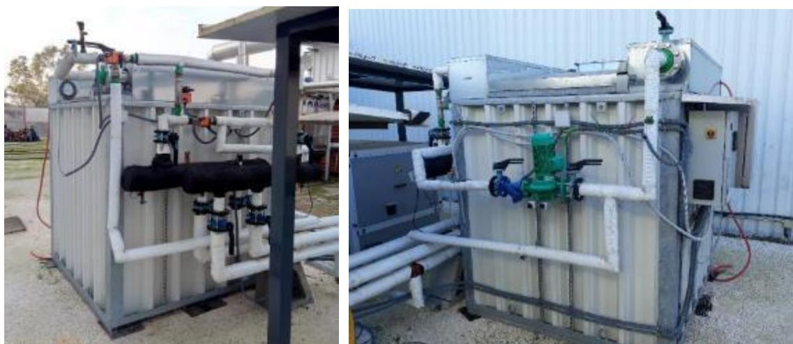
Figure 38. PCM tank with own hydraulics
