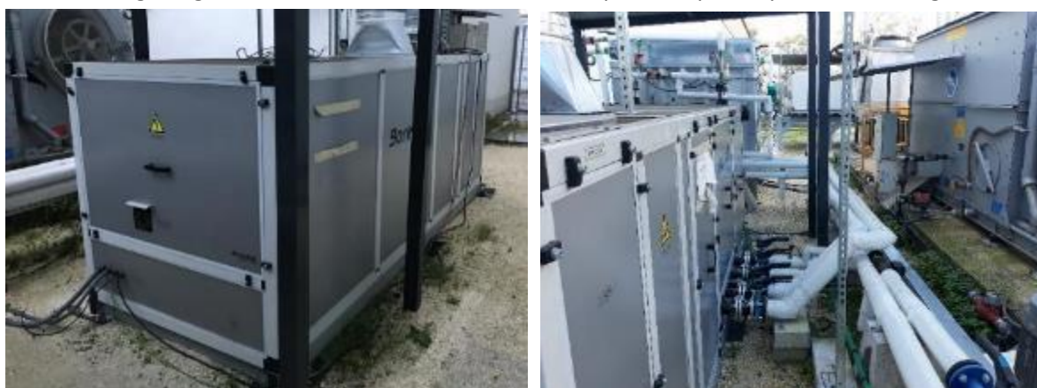
Figure 40. Borealis chiller with own hydraulics
