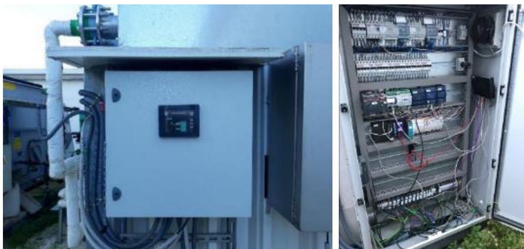
Figure 43. Fafco control cabinet and primary control cabinet
