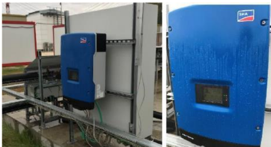
Figure 36. PV inverter
