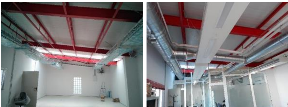
Figure 48. Chilled Beams during installation
