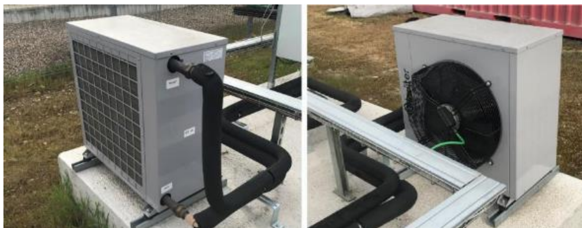
Figure 35. Dry cooler of the PVT system
