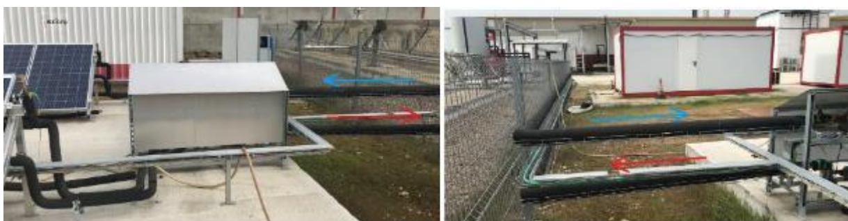
Figure 33. Supply and return water pipes from the solar field to stratified tank
