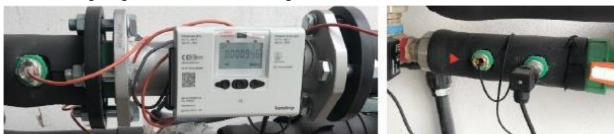
Figure 52. Flow rate meter and temperature and pressure sensor in the radiant floor system
