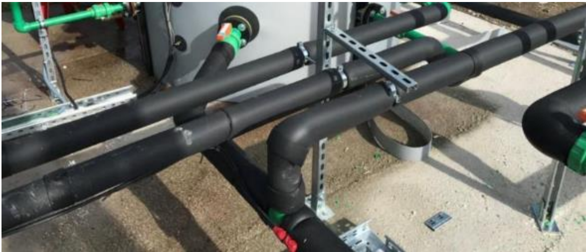
Figure 22. Pipes with insulation
