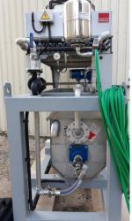
Figure 8 and Figure 9. Image of heat exchanger, installed in the pilot of Madrid (front view).
