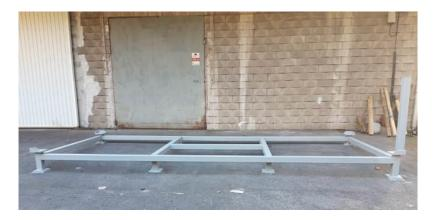
Figure 27. Structure prepared to receive the HP-LowUp container.
