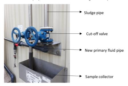
Figure 6. Detail of the system's connection to the bio digester reactor.
