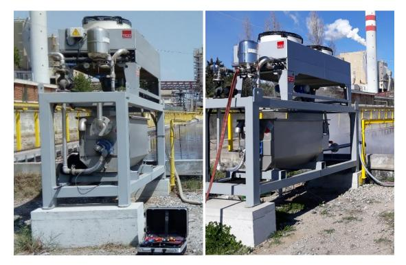
Figure 17. Heat recovery system and auxiliary systems after their installation in Setubal.
