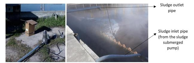
Figure 16. Sludge pump before been submerged (left side) and sludge pump connection (right side).
