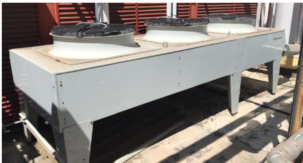
Figure 18. Dry cooler installed in Seville demo
