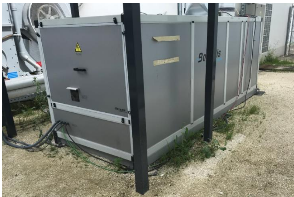
Figure 22. AHU & CHILLER installed in Seville demo
