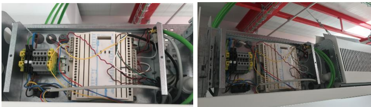
Figure 82. Control panel in the chilled beam.
