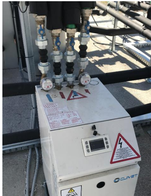
Figure 60. Heat pump connections and security components.
