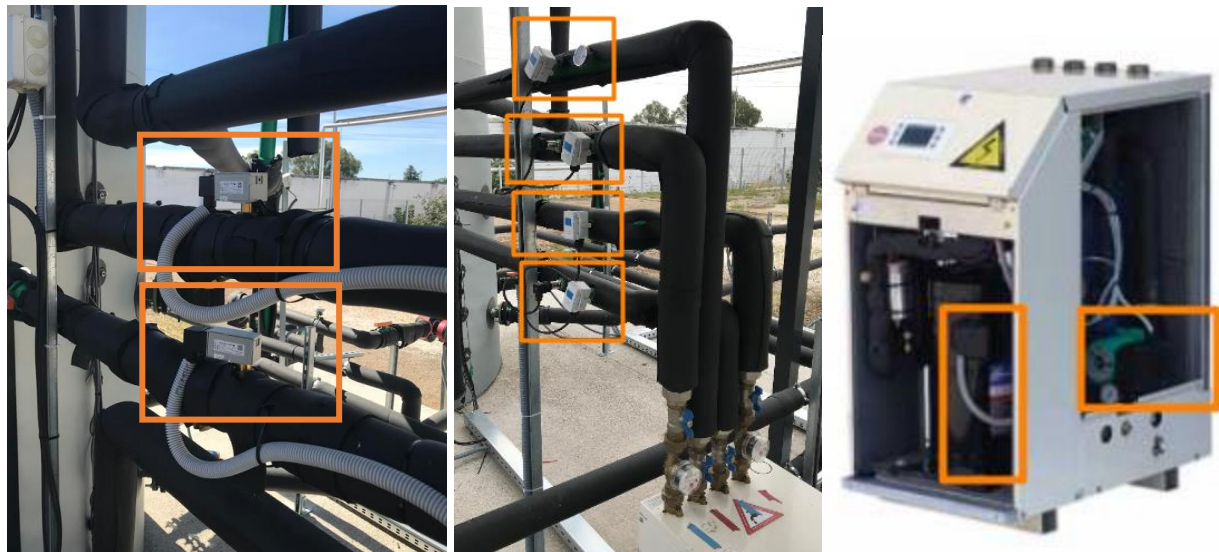
Figure 61. Control and security components installed in the heat pump.
