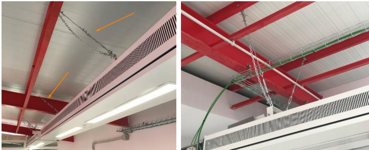
Figure 80. Hanging system of chilled beams.
