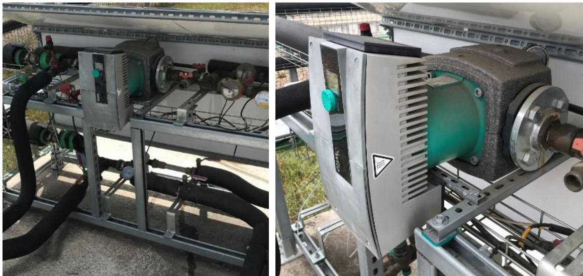
Figure 50. Detail of solar field pump.
