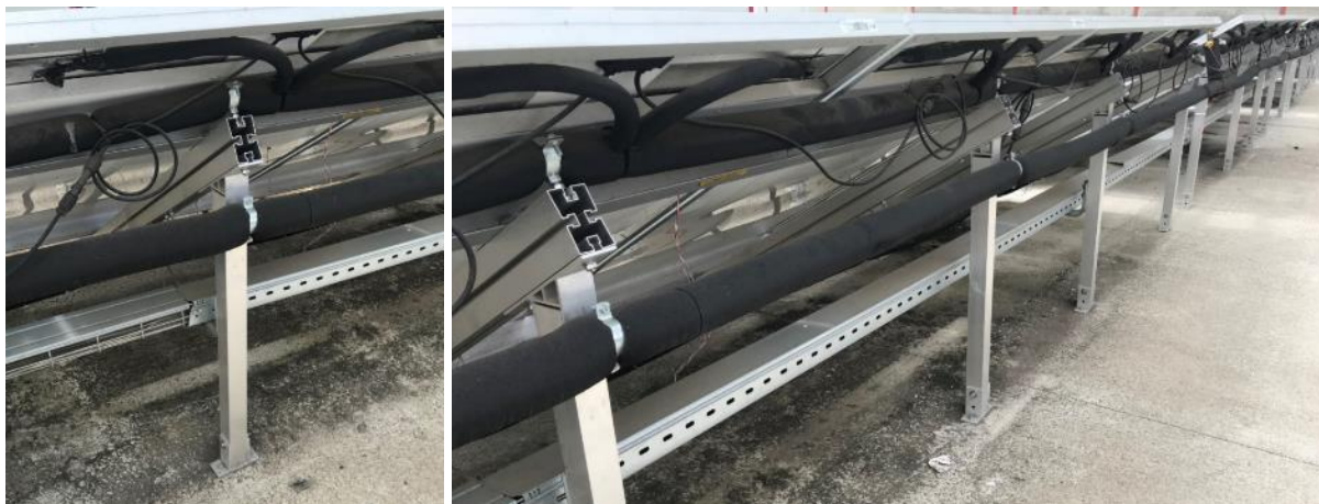
Figure 45. Panel bearing structure.
