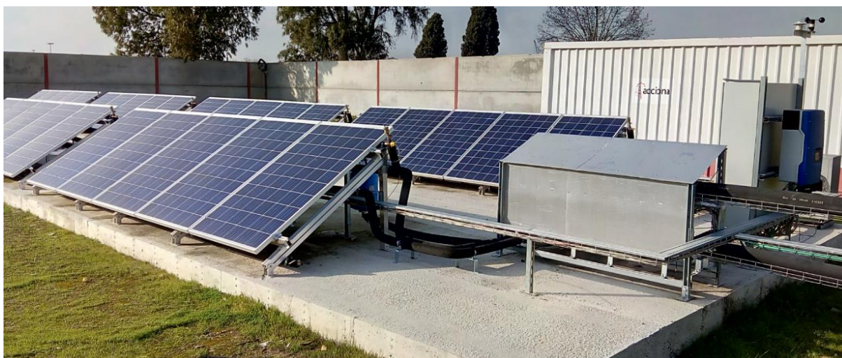
Figure 2: Heating system – Solar field with the pumping station
