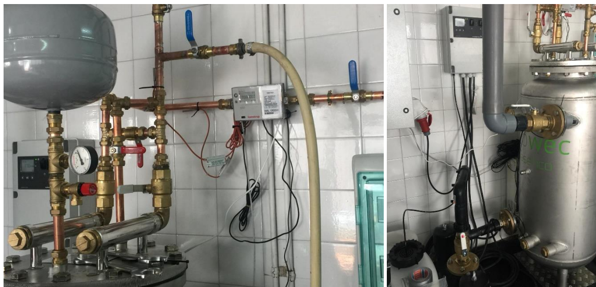
Figure 70. Grease separator-pumping station-recovery tank.
