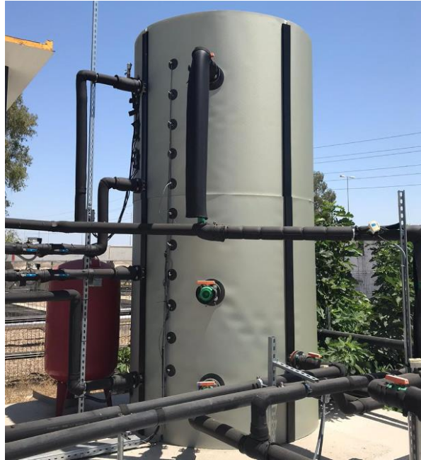
Figure 6. Stratified tank installed in Seville demo
