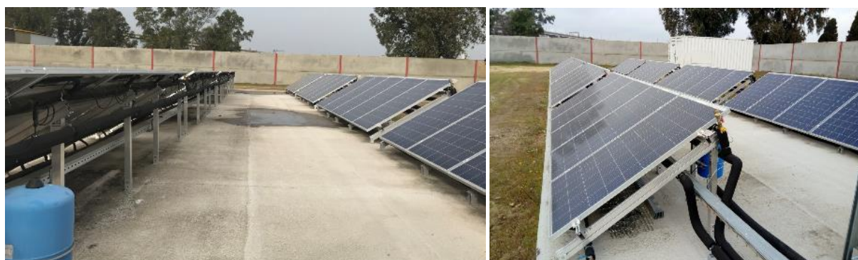
Figure 44. Free space between strings of panels.
