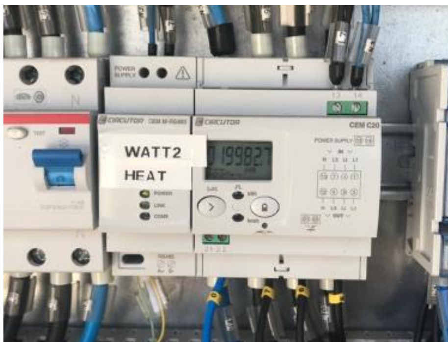
Figure 38. One of the electrical energy meters installed in Seville demo
