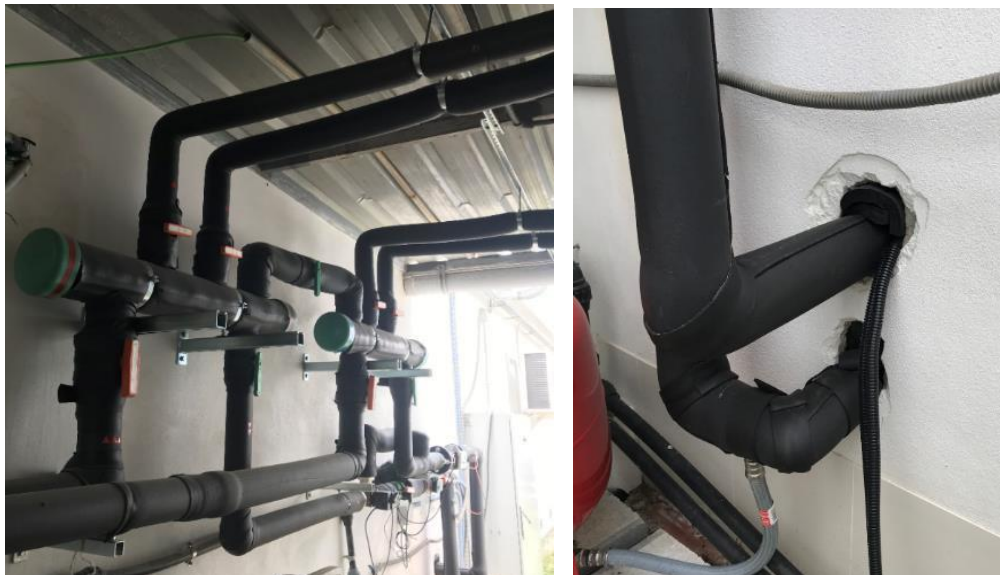
Figure 65. Supply and return manifold (left), supply and return pipes through the wall to the radiant floor.
