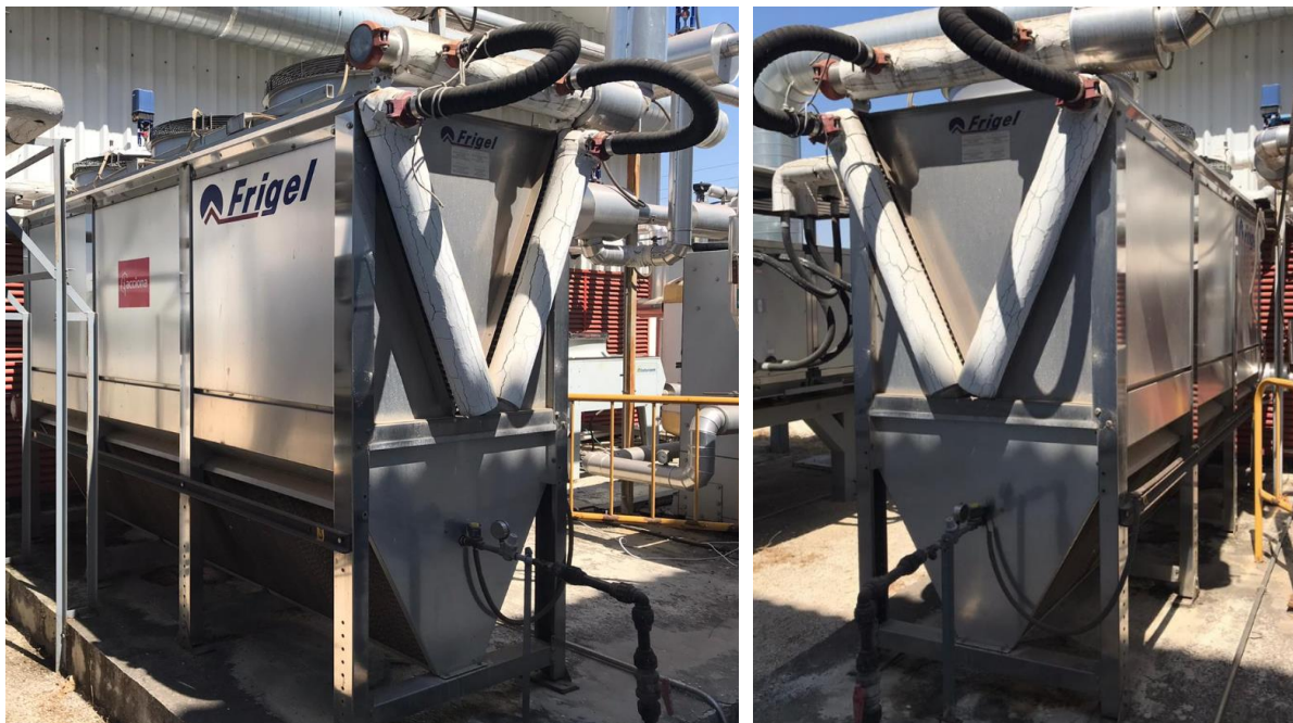
Figure 34. Cooling tower installed in Seville demo
