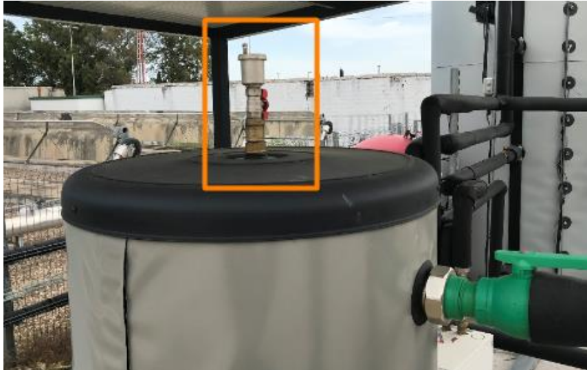
Figure 73. Bleeder on Wasenco Tank.
