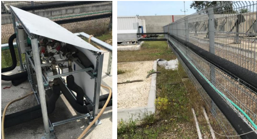
Figure 53. Structure to avoid sun radiation (left) and anchorages of solar field pipes.
