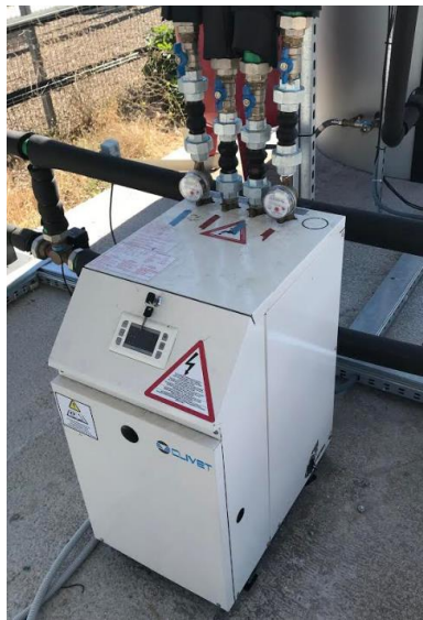
Figure 12. Heat pump installed in Seville demo
