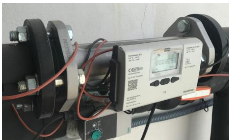
Figure 39. One of the flow meters installed at Seville demo
