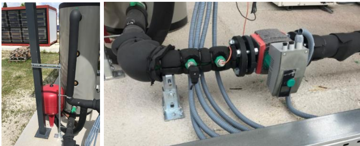
Figure 72. Fixing structure to hold pipes, pump and tank in Wasenco emulator.
