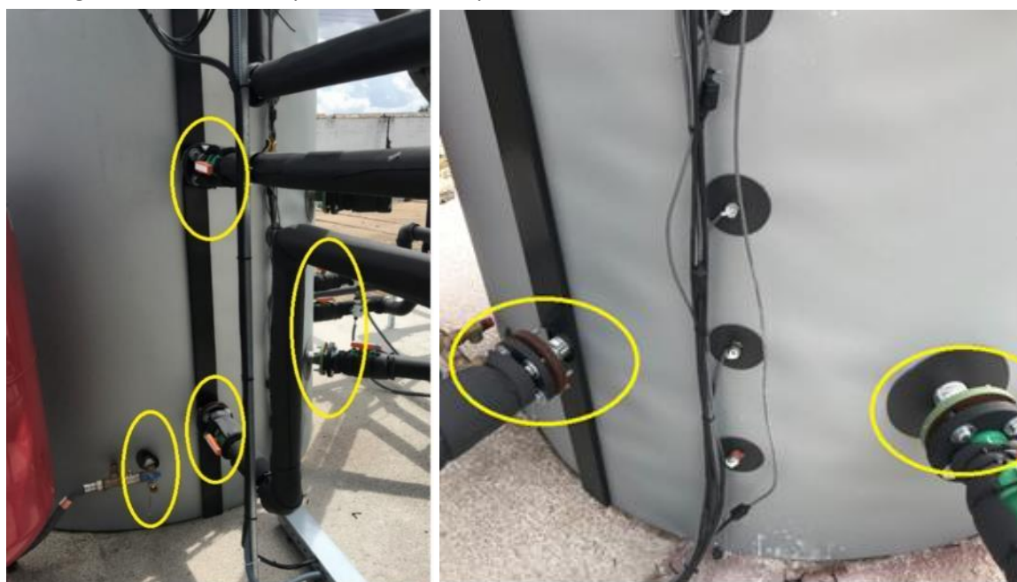
Figure 55. Joints and pipes connections on the storage tank.
