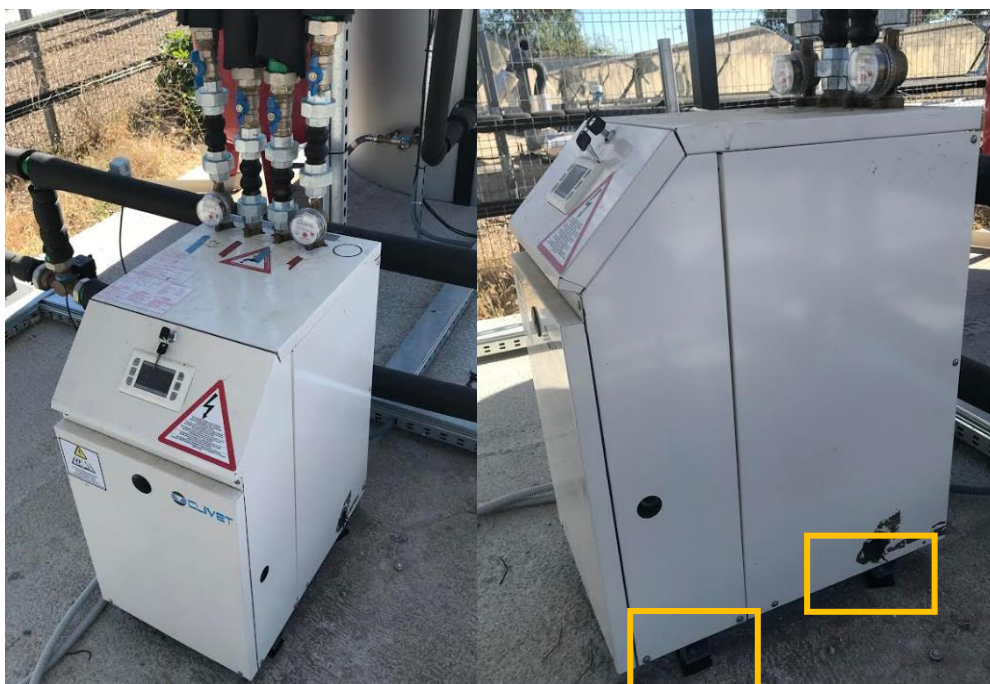
Figure 59. Supporting recommended of the heat pump.
