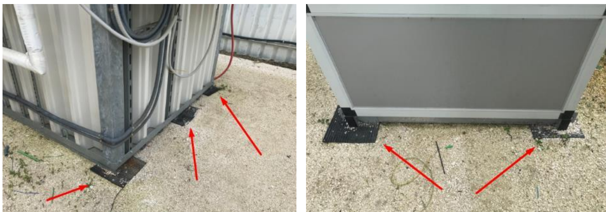
Figure 77. Rubber sheets in PCM Tank and Chiller.
