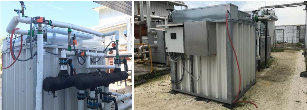
Figure 25. PCM tank installed in Seville Demo
