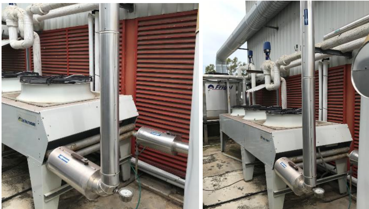
Figure 76. Insulation pipes and joints in a dry cooler.
