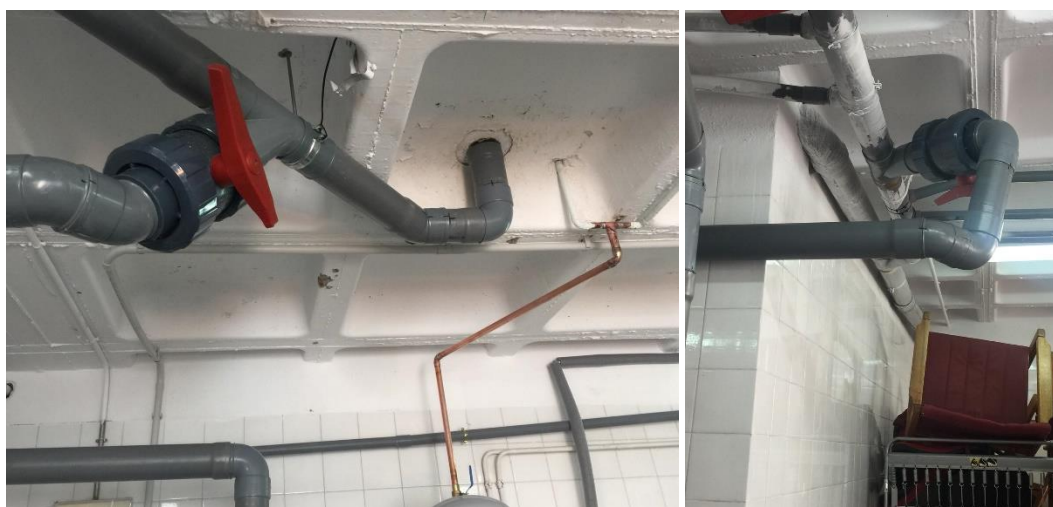
Figure 68. waste water bypasses
