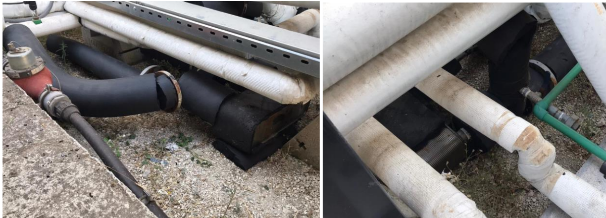
Figure 37. Heat exchanger between cooling tower and return from chilled beams
