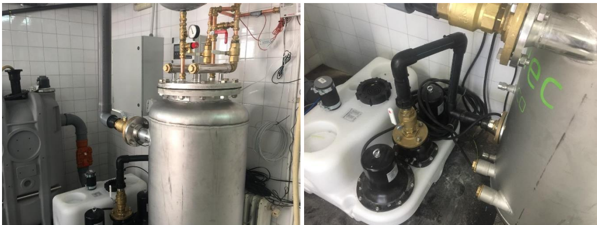
Figure 69. Grease separator-pumping station-recovery tank.
