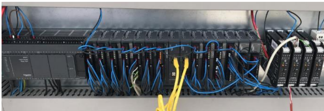
Figure 49. Control connections of local plc.
