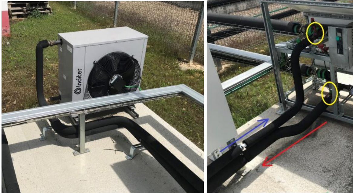
Figure 47. Dry cooler (left) and temperature sensor for the dry cooling system.
