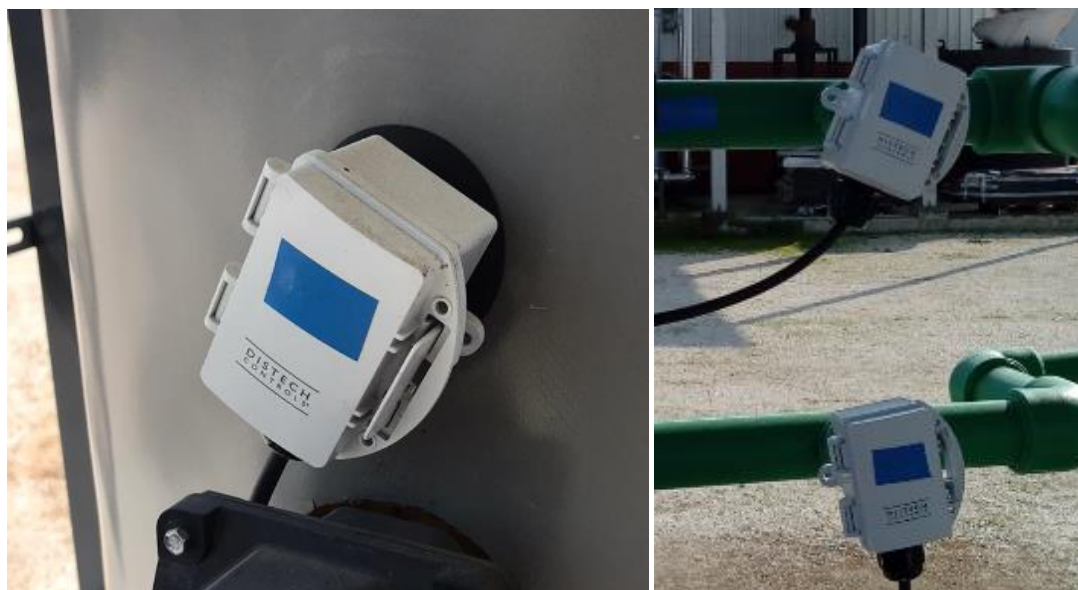
Figure 42. Few of the temperature sensors installed in Seville demo
