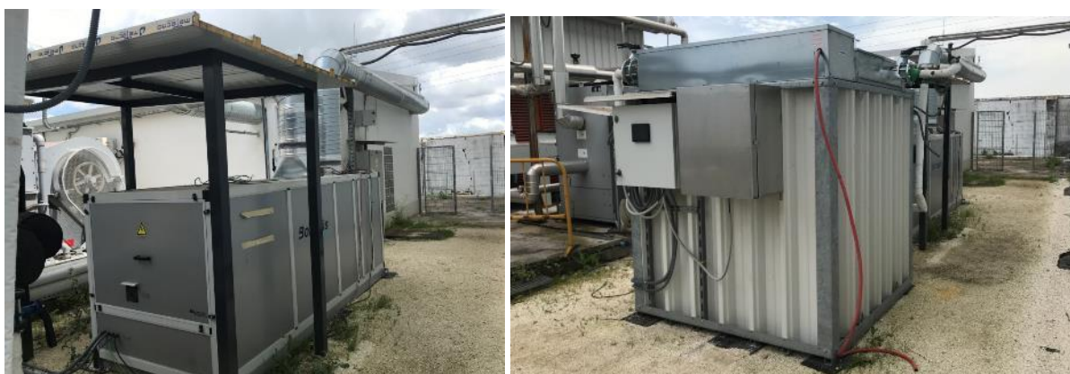
Figure 78. Free space around PCM Tank and Chiller.
