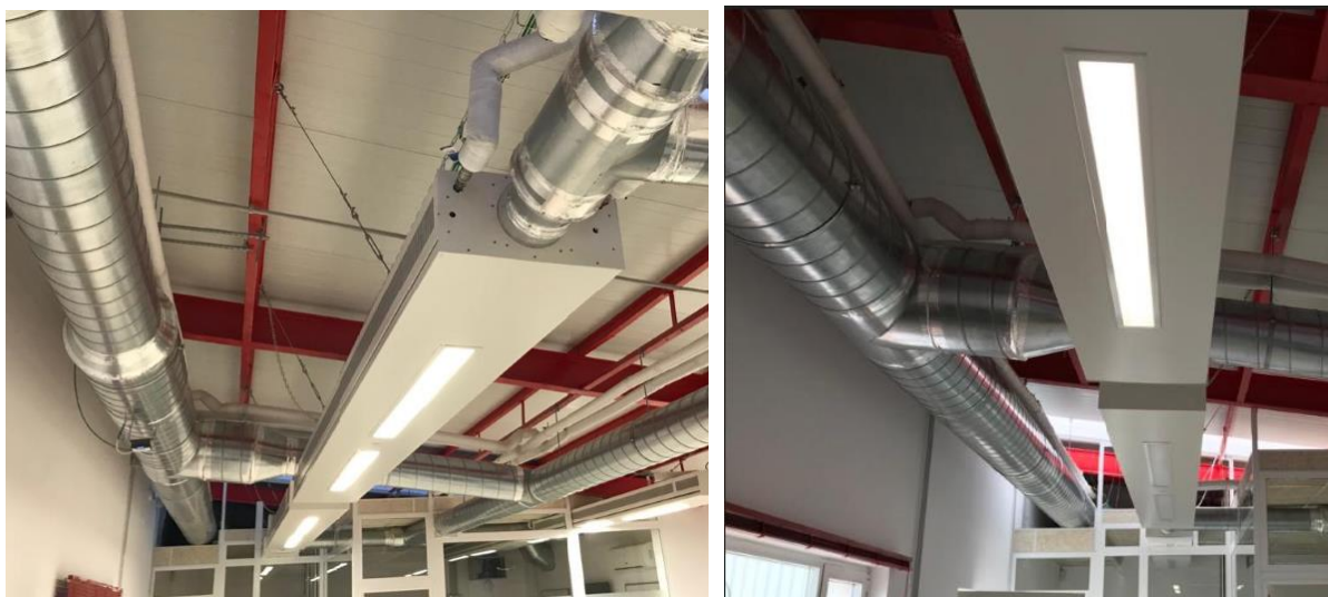
Figure 31. Chilled beams installed inside the office
