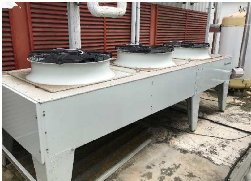
Figure 74. Free recommended space around the dry cooler.
