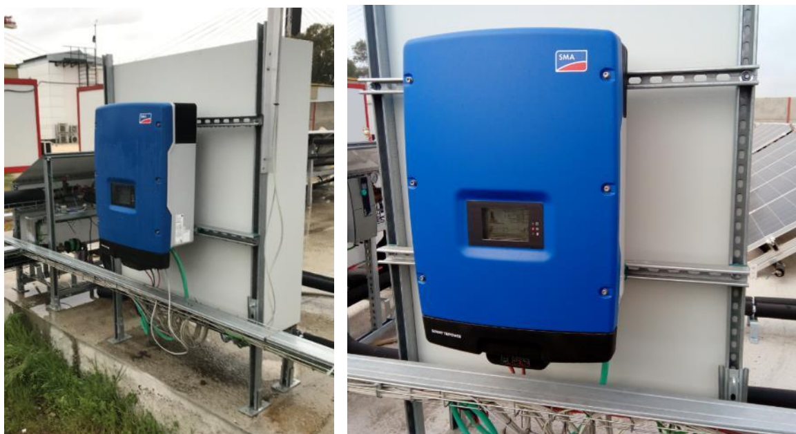
Figure 54. Structure for DC/AC Inverter.
