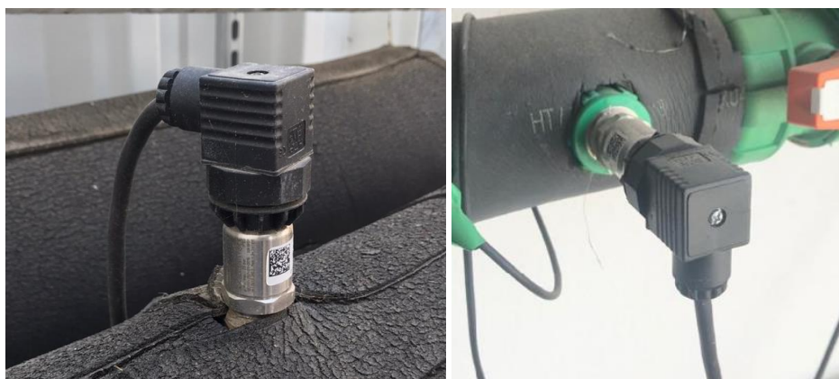
Figure 40. One of the pressure sensors installed in the Seville demo
