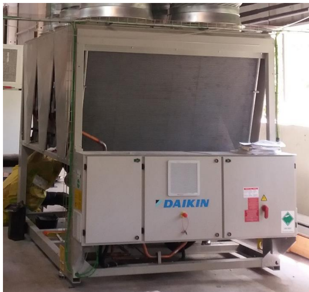
Figure 31: Chiller installed in Tecnia thermal lab
