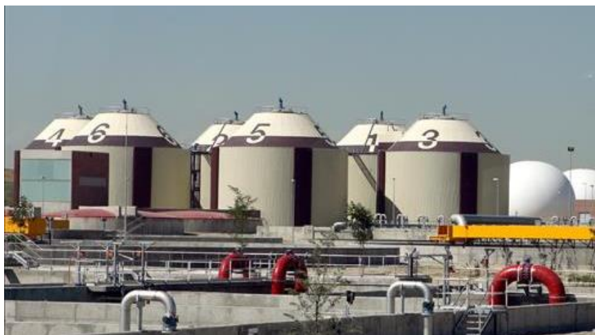
Figure 3: Anaerobic digester in EDAR Arroyo Culebro Cuenca Baja
