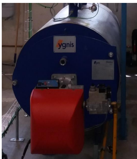
Figure 30: Boiler installed in Tecnia thermal lab
