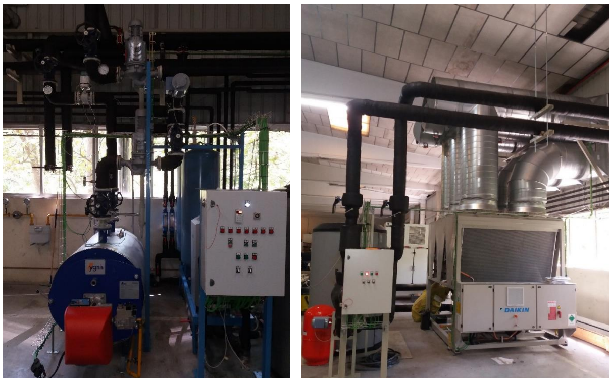
Figure 33: Pipe network of the boiler and chiller systems before HP integration
