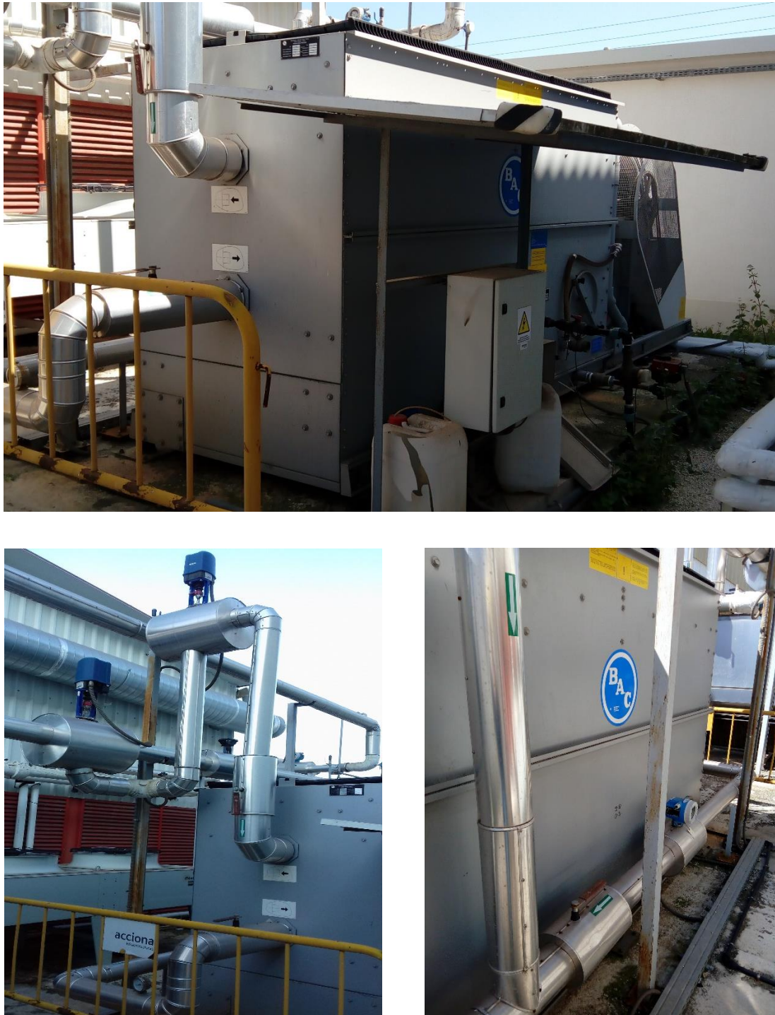
Figure 34: Cooling Tower
