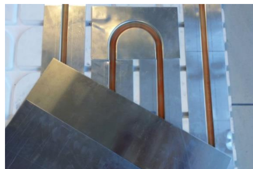
Figure 8: Radiant floor
