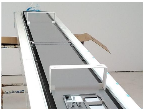
Figure 32: Chilled beam anchoring points detail
