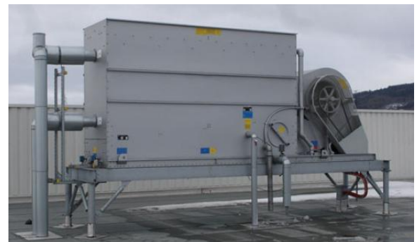
Figure 17: Cooling tower
