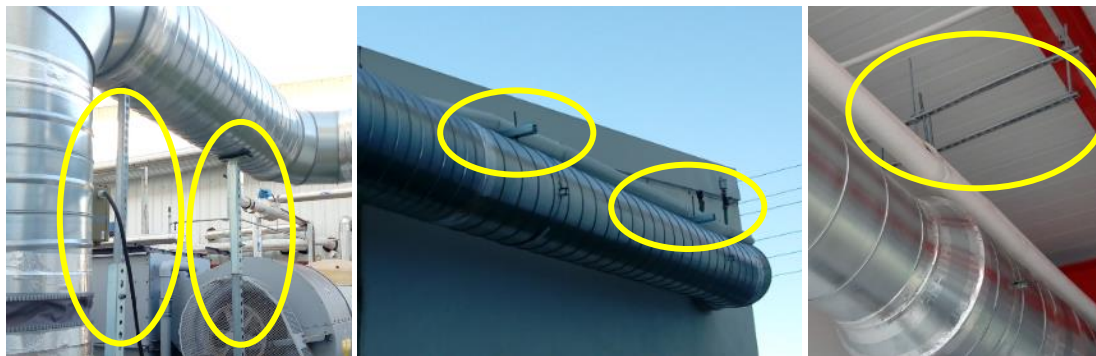
Figure 11. Anchoring of the air duct
