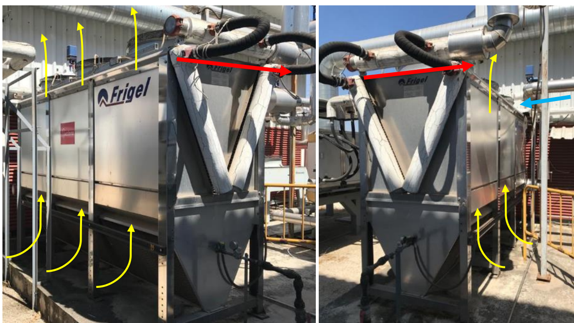
Figure 24. Inlet water manifold (blue), Outlet water manifold (red), direction of air flow (yellow)
