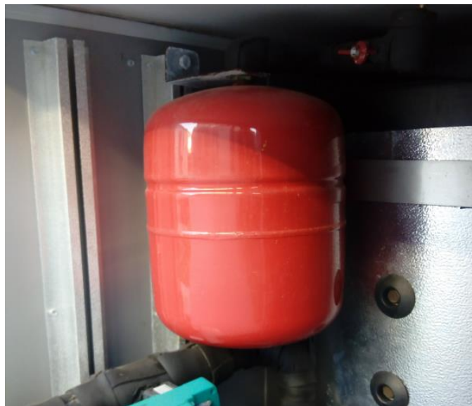
Figure 9. Expansion vessel
