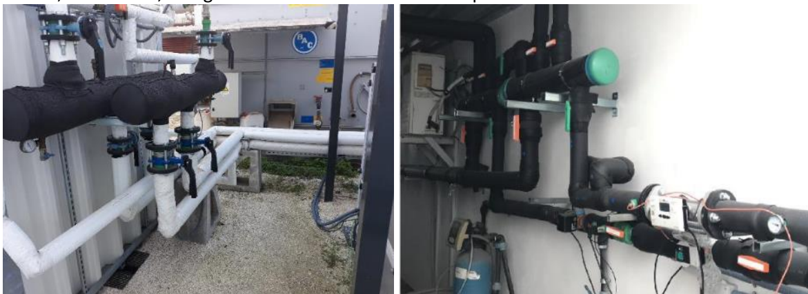
Figure 12. Isolating of different element in the installation
