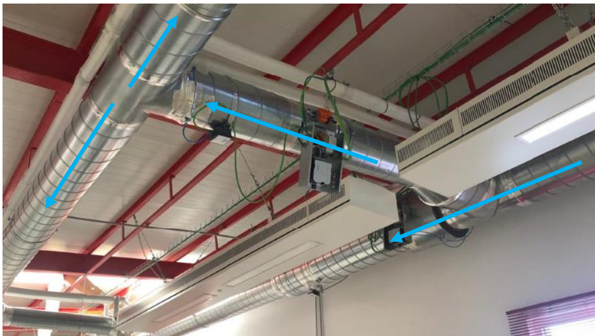
Figure 23. Air duct with direction of the air
