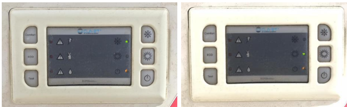
Figure 68. Integrated heat pump keypad. Cool mode (left) and Heat mode (right)
