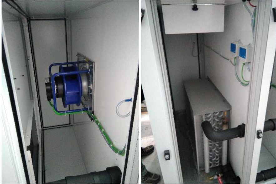
Figure 4. Plug fan and cooling coil
