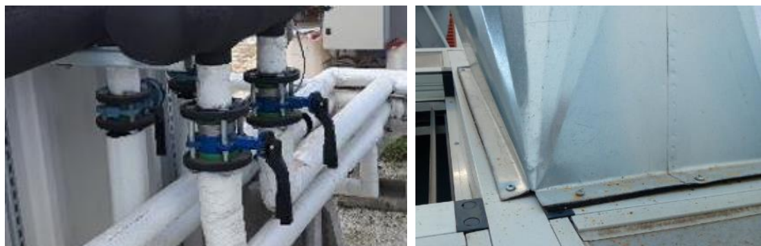
Figure 13. Joints in air and water circuit
