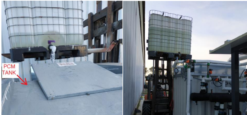
Figure 16. PCM tank filling
