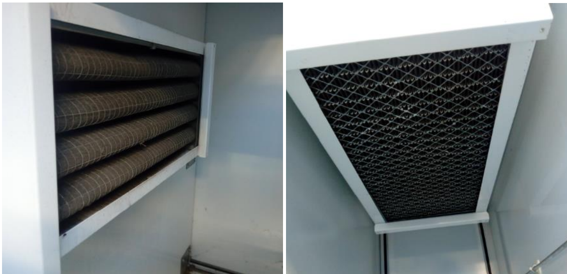
Figure 5. Filters inside the AHU
