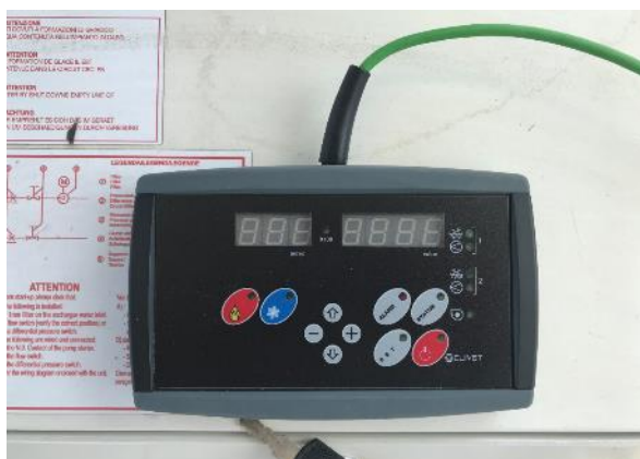
Figure 69. External heat pump keypad
