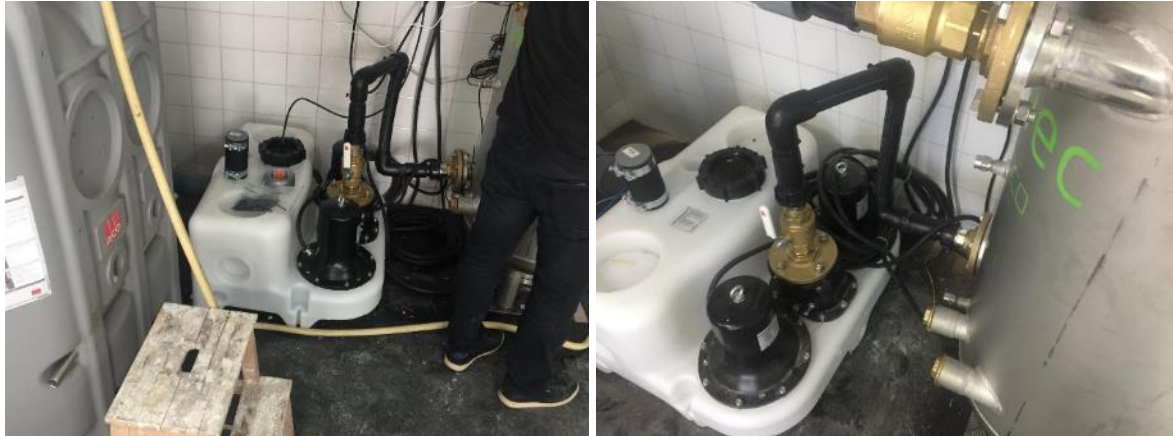
Figure 89. Pumping tank station
