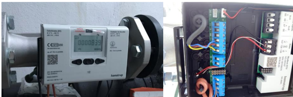
Figure 31. Connection of flow meter (electrical and network)
