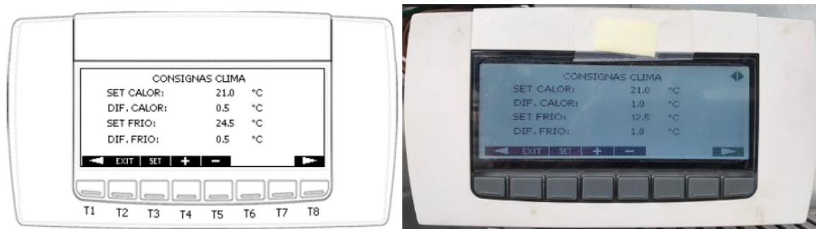
Figure 36. AHU setpoints
