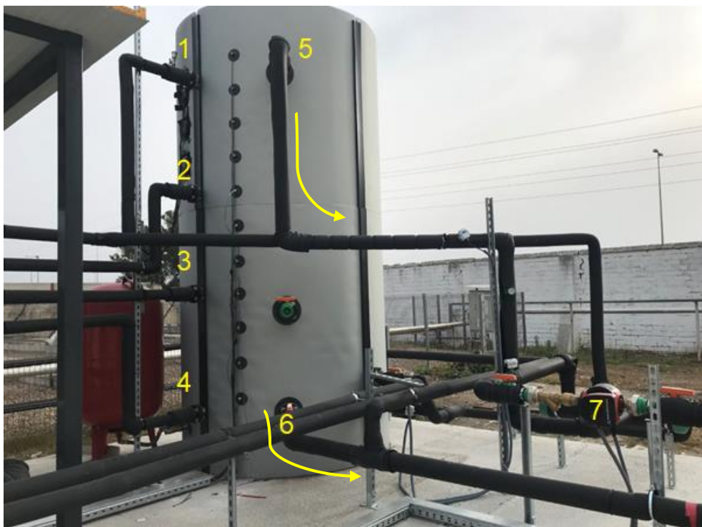
Figure 67. Connection of the stratified tank
