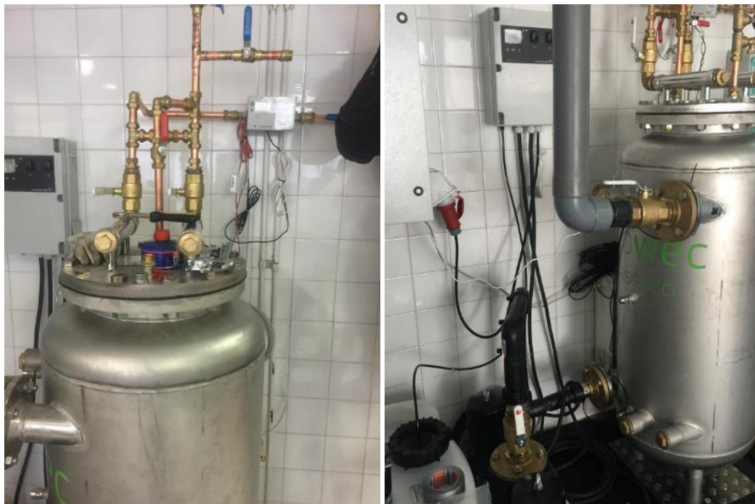
Figure 87. Connections of piping to tank
