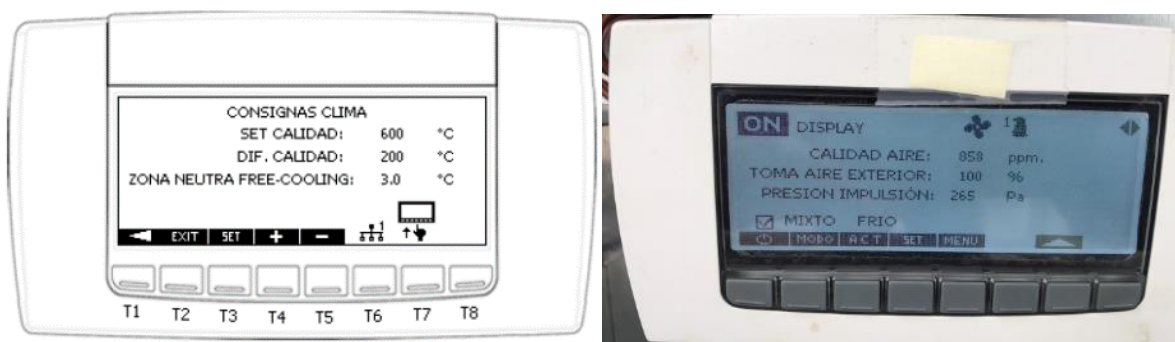
Figure 37. AHU setpoints
