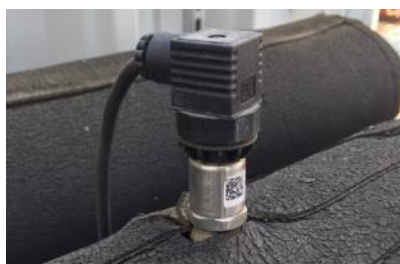
Figure 30. Pressure sensor
