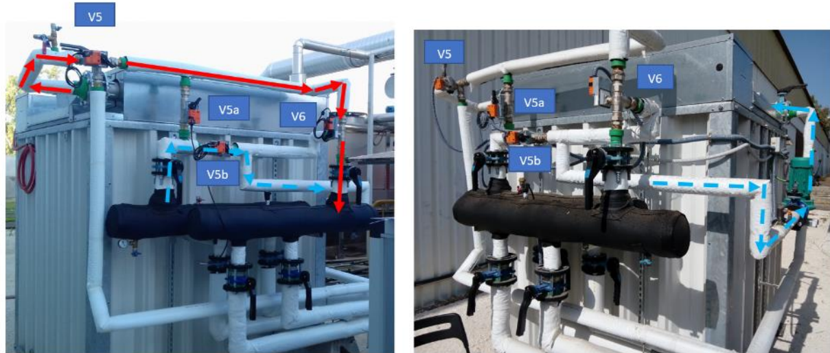
Figure 18. Position of valves in charge mode
