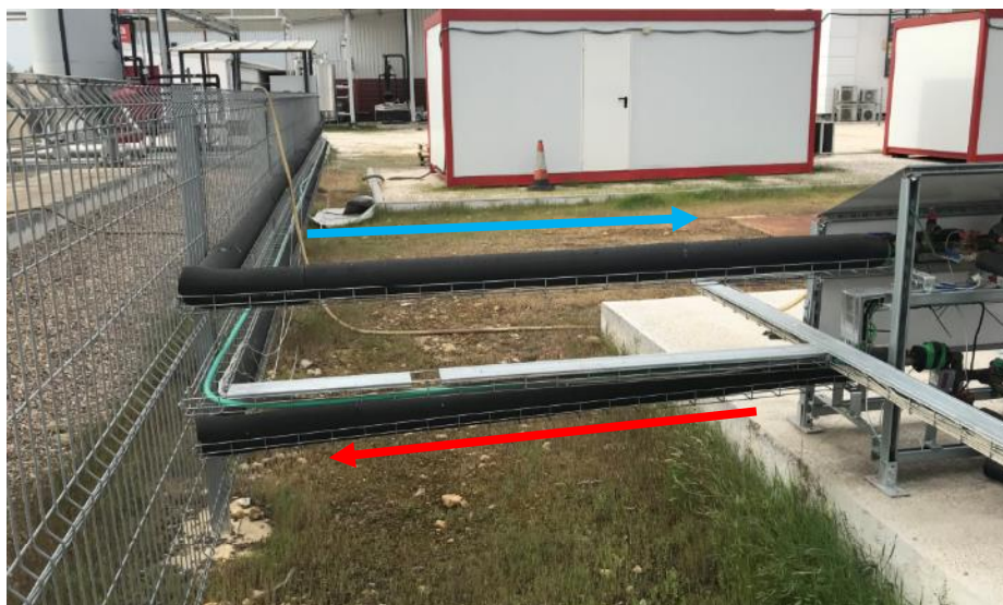
Figure 62. Inlet water (blue) and outlet water (red) in solar field
