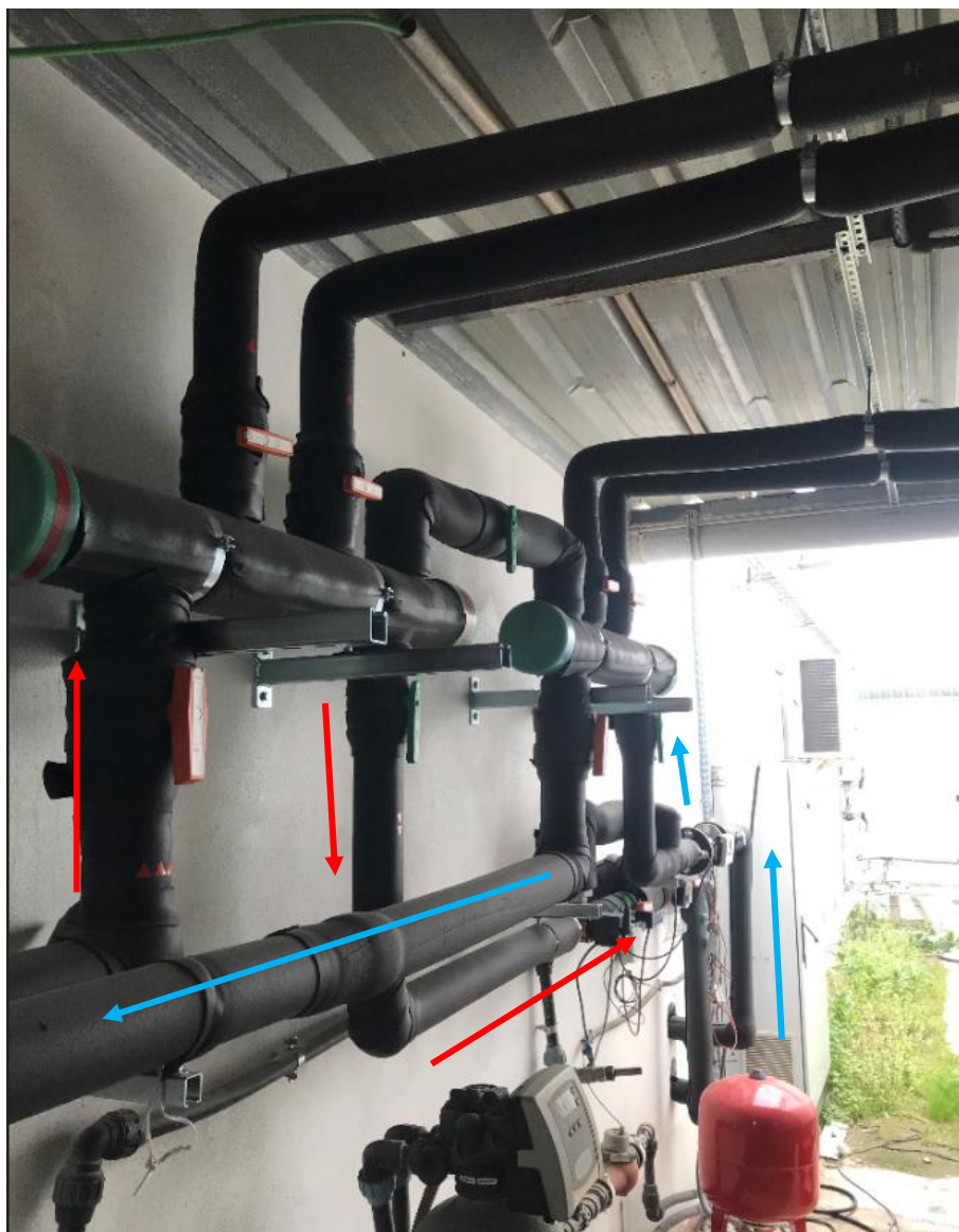
Figure 65. Schema of the radiant floor supply and return water
