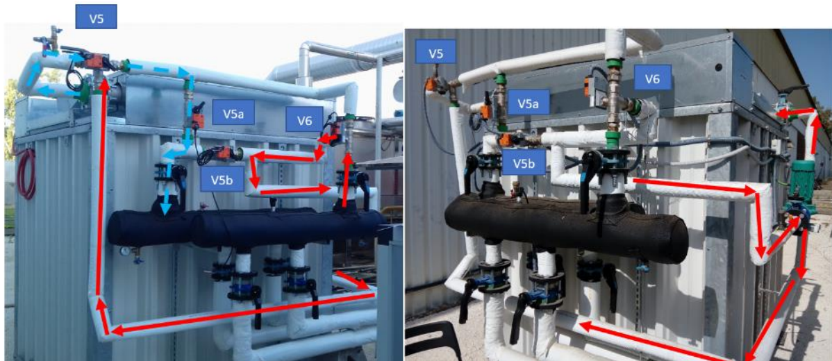
Figure 20. Position of valves in discharge mode
