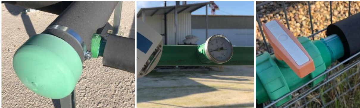
Figure 8. Different parts of the installation, PPR pipes and the isolation
