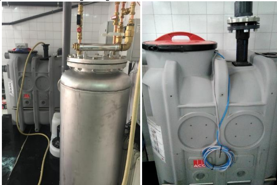
Figure 88. Grease tank
