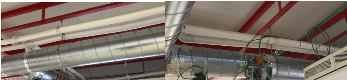
Figure 22. Some pipes of the hydraulic circuit
