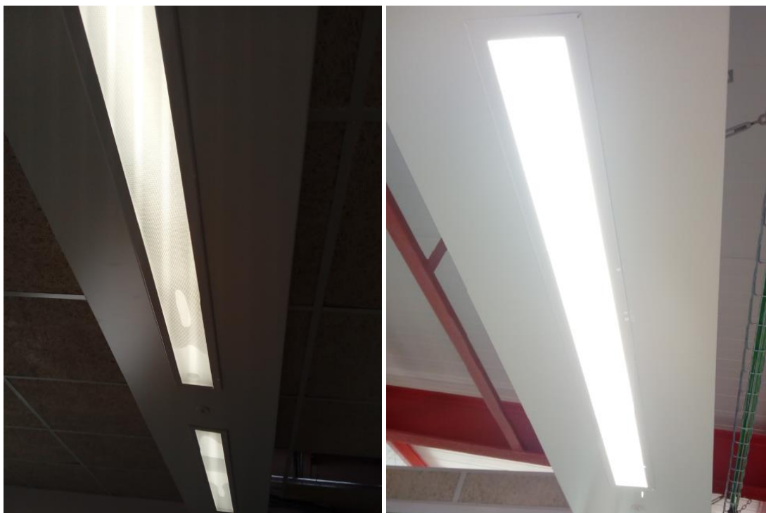
Figure 85. Condensation problems in chilled beams
