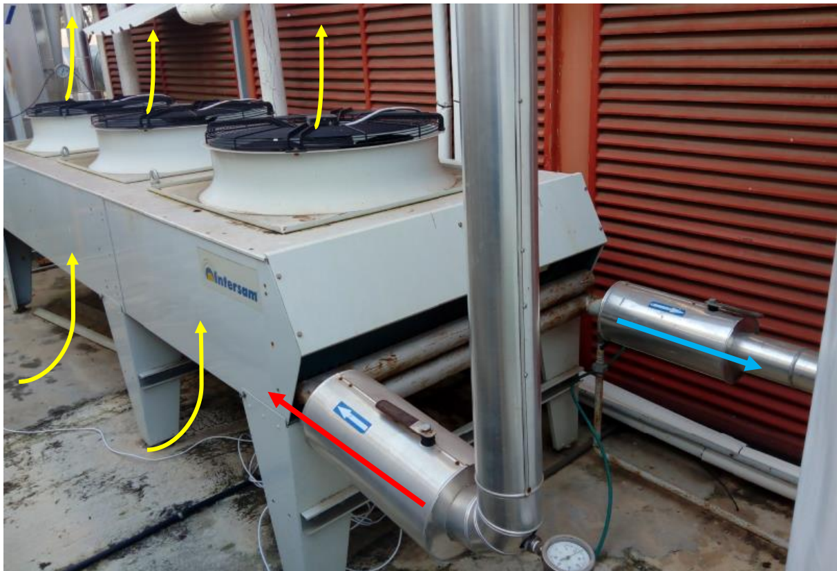
Figure 71. Water and air direction on the dry cooler. Inlet hot water (red arrow), outlet cold water (blue arrow) and air (Yellow arrow)
