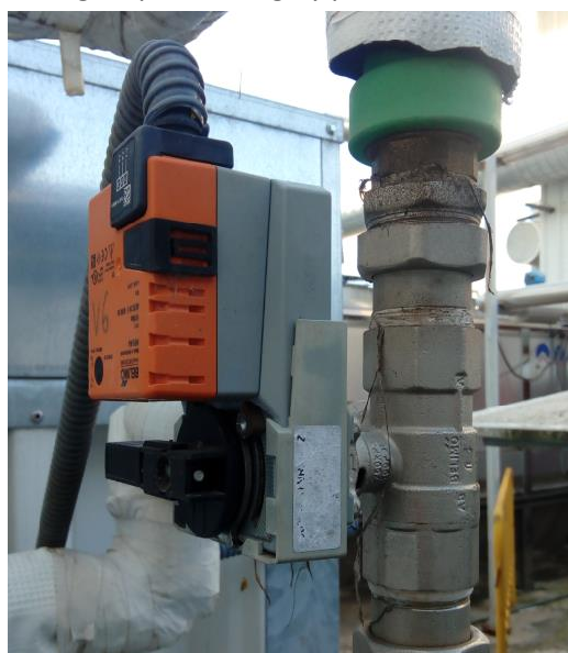
Figure 26. 3-ways valve with its actuator
