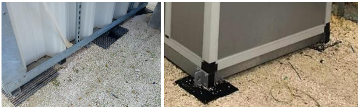
Figure 2. A type of unit support on the floor
