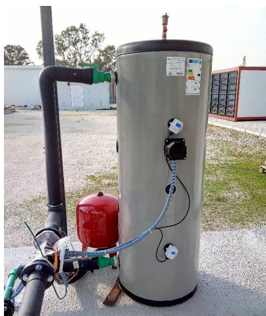
Figure 26: Integration of the thermal emulator (to represent the performance of the grey-energy heat-recovery system)
